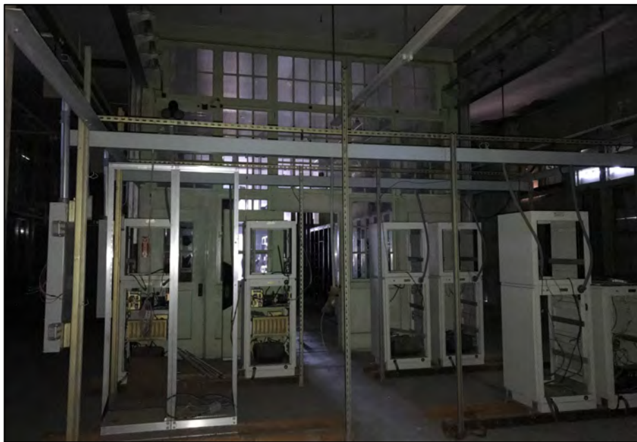
Photograph 9: Non-historic metal framing for removed communications equipment located south outside of central control room, camera facing north, July 17, 2018 (AECOM).
