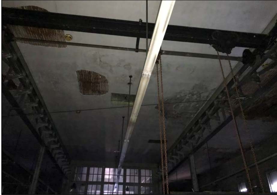
Photograph 12: Detail view of metal roof supports, metal track system, and damaged ceiling. Lights are not original, camera facing north, July 17, 2018 (AECOM).
