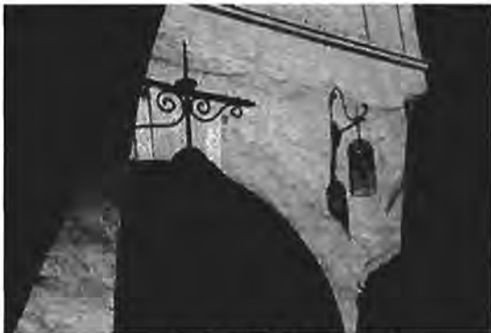
Detail of the south side of the front façade.
