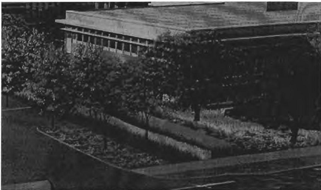
Detail at site entry - Channel viewed from above
