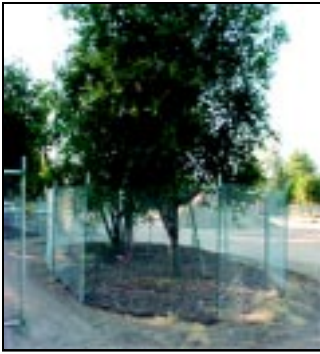
IMAGE 2.15-1 Tree Protection Fence at the Dripline
