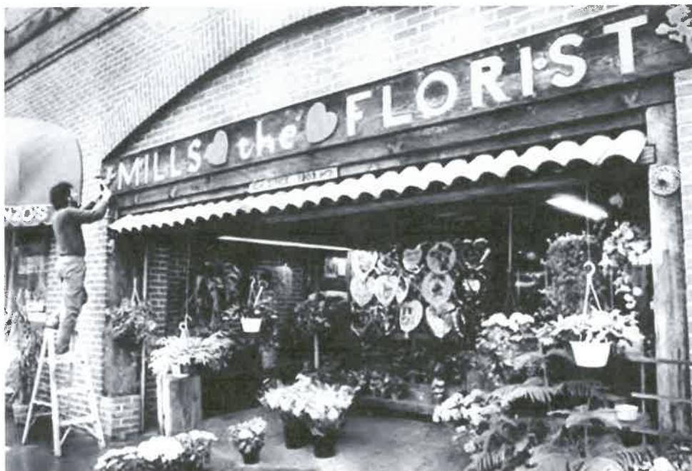
Figure 5. Storefront of 235 University Avenue following major façade alteration, 1980s. Source: Palo Alto Historical Association Photograph Collection, #092-088.
