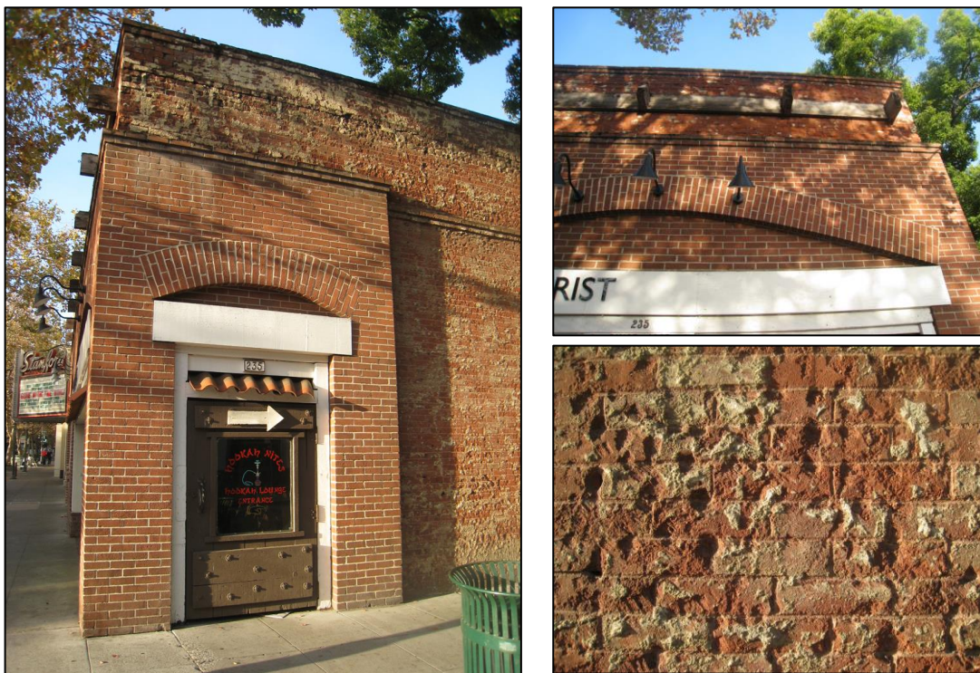
Figure 12: New brick façade added to original brick structure, visible at northeast corner (left) and front elevation (top right); original brickwork visible on the lateral elevation (bottom right).
