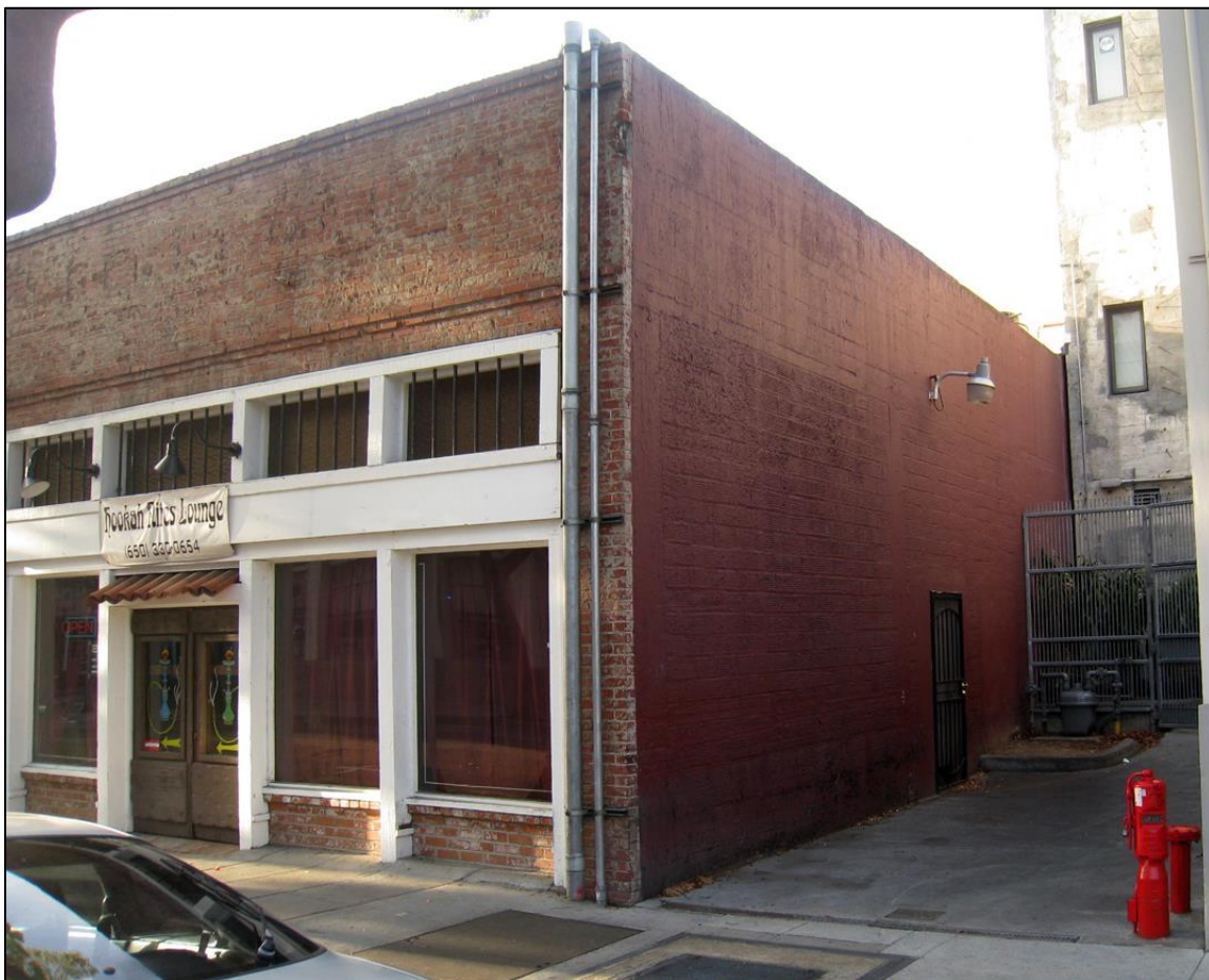
Figure 5: Lateral and rear elevation, view facing south
