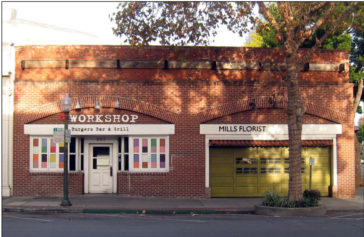
Figure 2: Front elevation, view facing northwest
