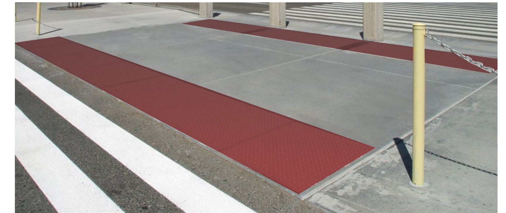
Flush Curb/ Truncated Domes
