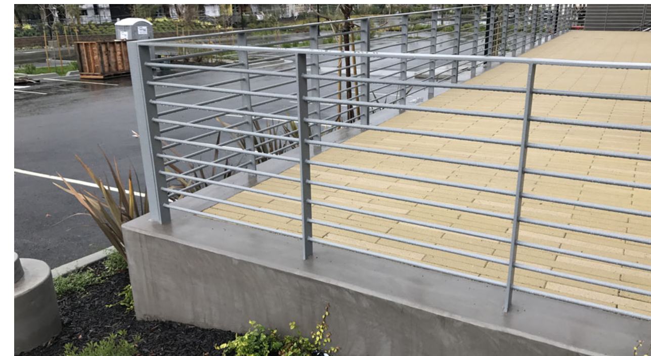
Concrete Retaining Wall & Guardrail
