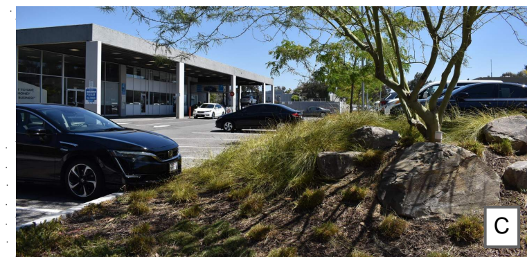
VIEW OF HONDA SERVICE RECEPTION CANOPY AND SHOWROOM
