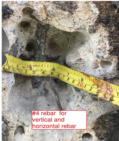
Rebar size for S1 location
