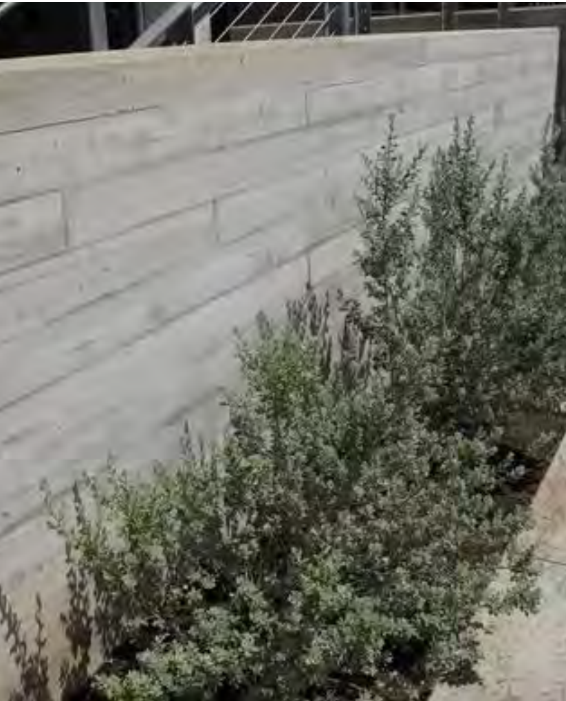
SE-2 BOARD-FORM CONCRETE WALL
