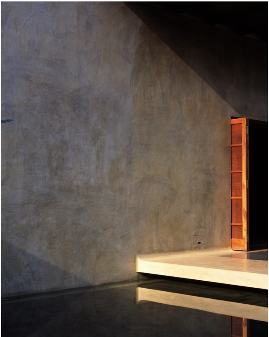
HIGH-QUALITY MATERIALS: SMOOTH-TROWELED PLASTER WALLS, WOOD SOFFIT, BOARD-FORMED CONCRETE, PAINTED METAL PLATE, FLOOR-TO-CEILING CURTAIN WALL
