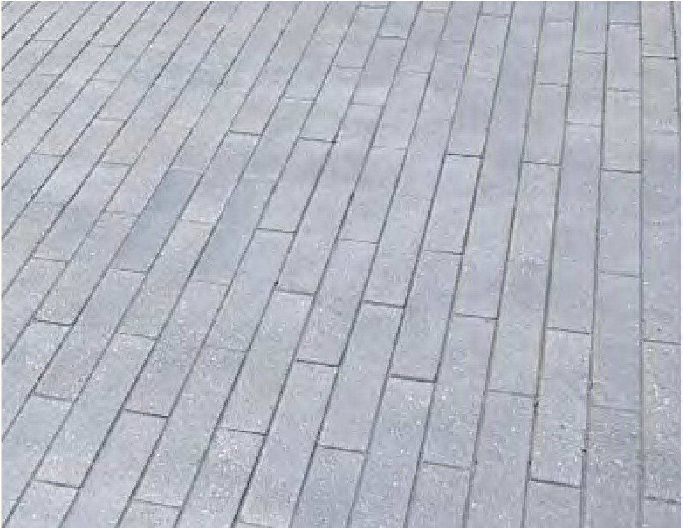
SM-2 SMALL CONCRETE UNIT PAVER
