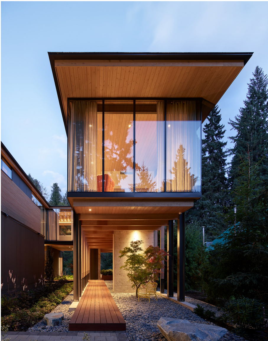
SOLAR CONTROL: DEEP ROOF PROJECTIONS AND MOTORIZED EXTERIOR ROLLER SHADES
