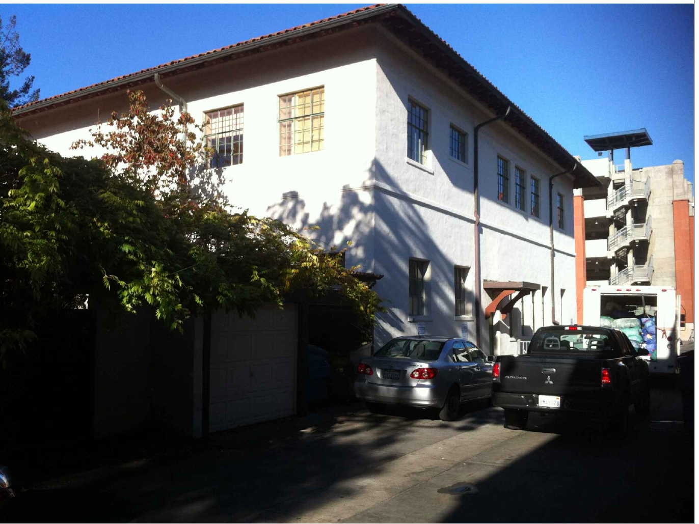
SOUTHWEST ELEVATION (BACK ALLEY)
