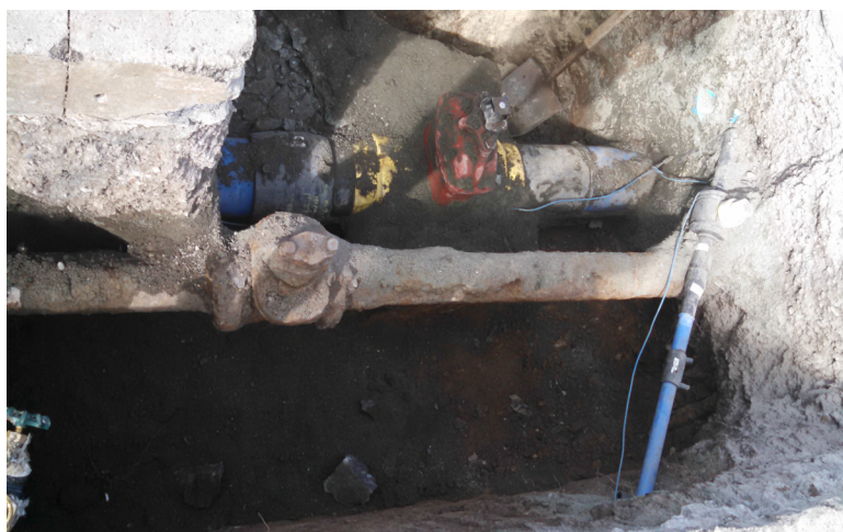
Installed 16" HDPE pipe waiting to be backfilled
