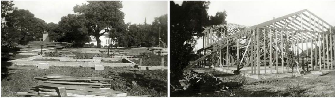
Figure 16: Construction photos for the Palo Alto Junior Museum and Zoo building. Source: Palo Alto Historical Association.
