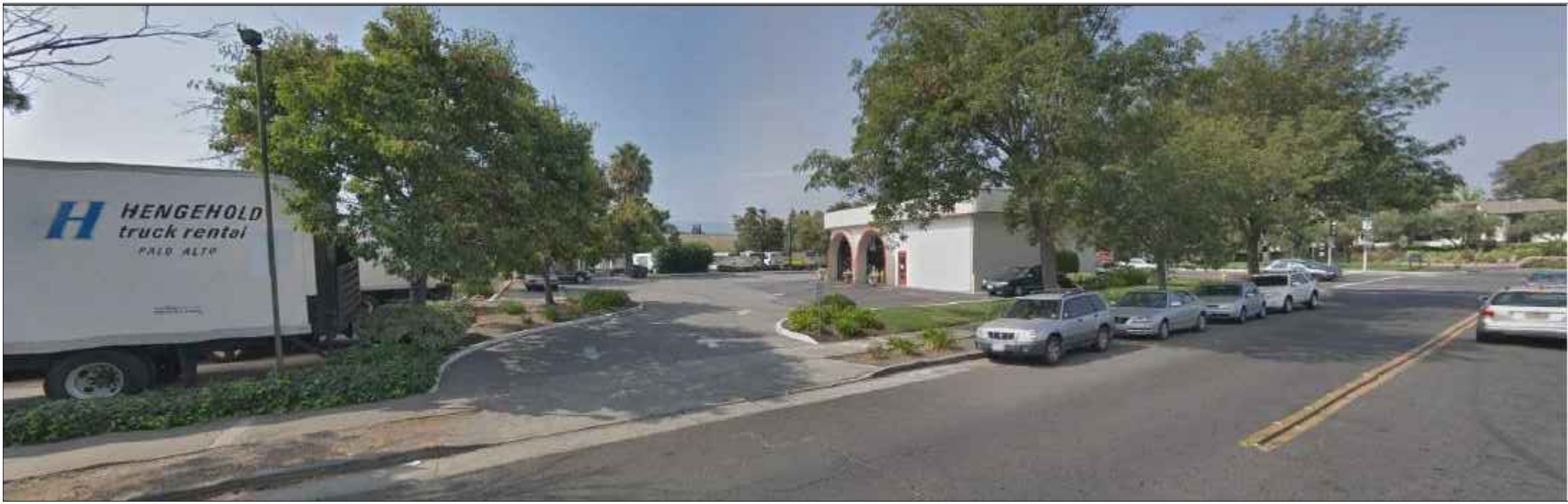
5. 780 SAN ANTONIO ROAD, PALO ALTO
