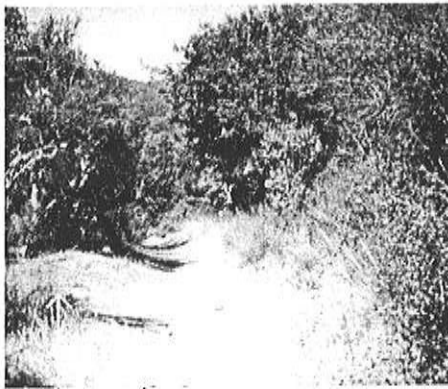
└ Entrenched Tread └ Berm of Displaced Soil
