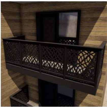
7 STEEL BALCONY RAILINGS WITH PARASOLEIL PANEL INFILL - BLACK MAGIC
