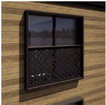
6 ALUMINUM GUEST ROOM GLAZING SYSTEM WITH PARASOLEIL SCREEN PANELS AND EXTENDED FACE CAPS
