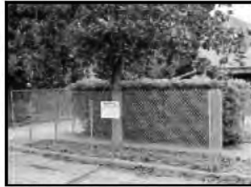
IMAGE 2.15-3 Tree Protection within a Planter Strip
