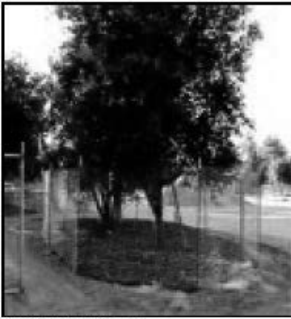
IMAGE 2.15-1 Tree Protection Fence at the Dripline
