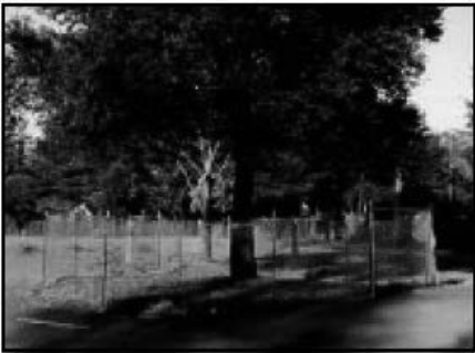
IMAGE 2.15-2 Tree Protection Fence at the Dripline
