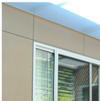
3 FORM CLADDING ON WALLS OF SECOND AND THIRD FLOOR
