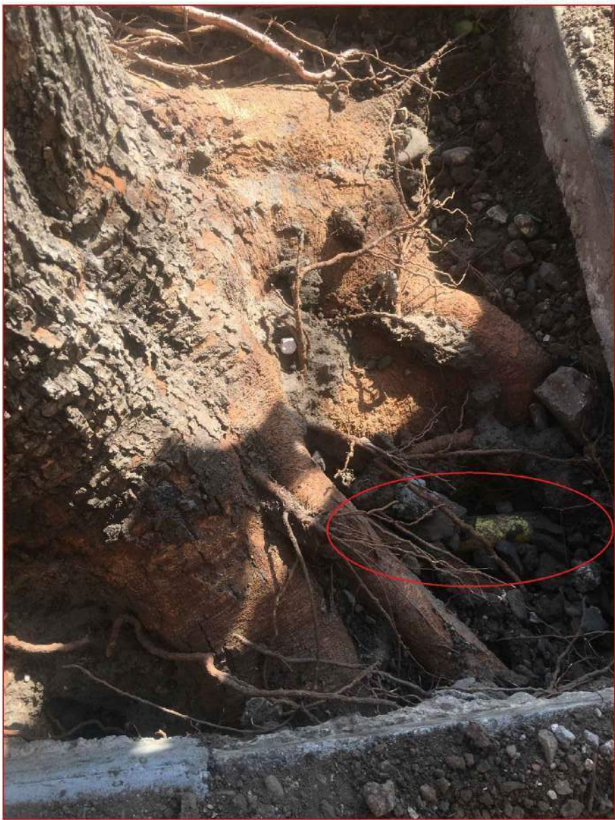
The above photo (Tree ID #1) shows a utility conduit line running under the roots along the building side of the trunk.
