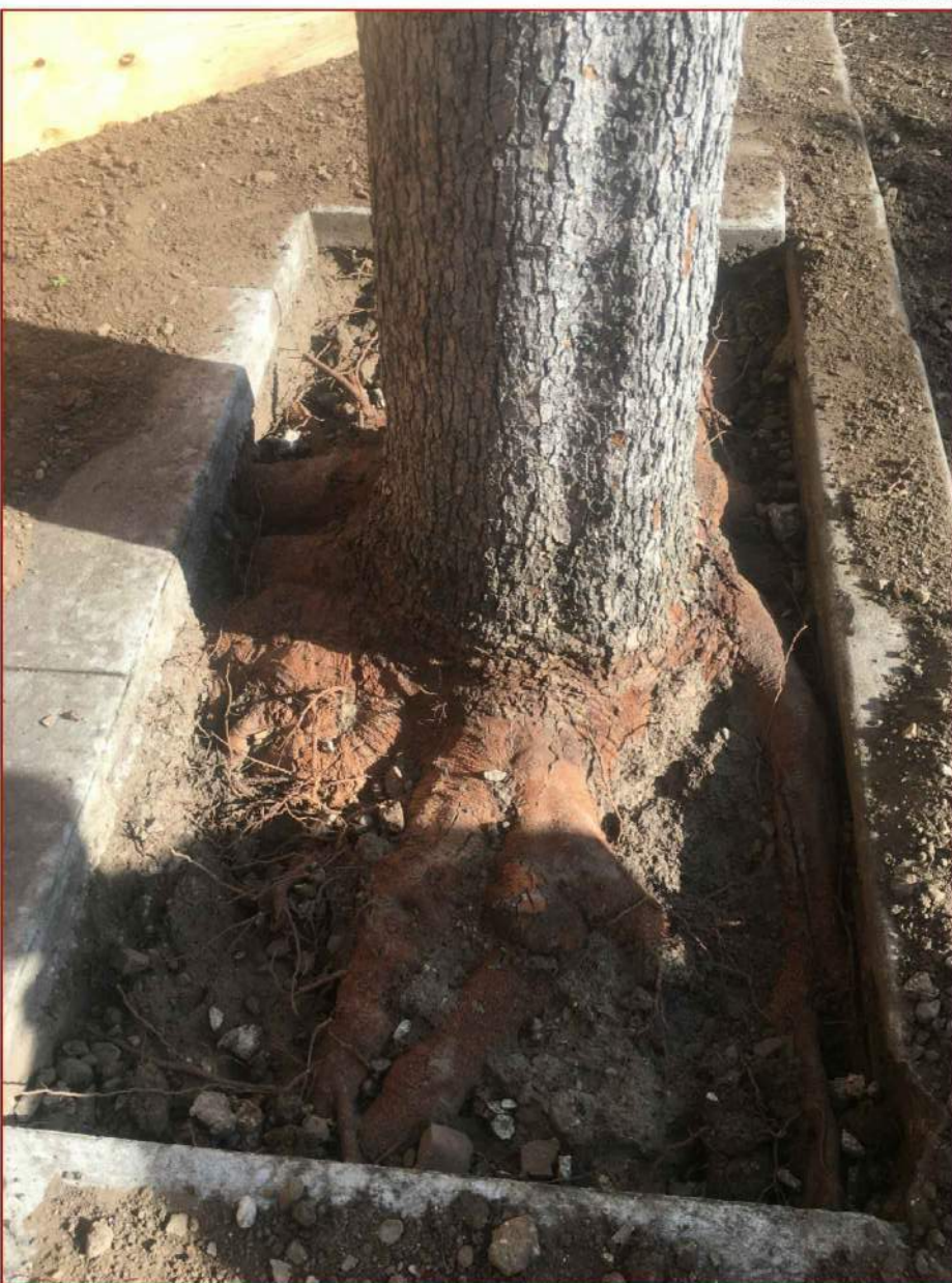
Tree ID #3 is shown in the photo above after it was excavated. Along the left side of this photo, three large roots 6" in diameter are visible.
