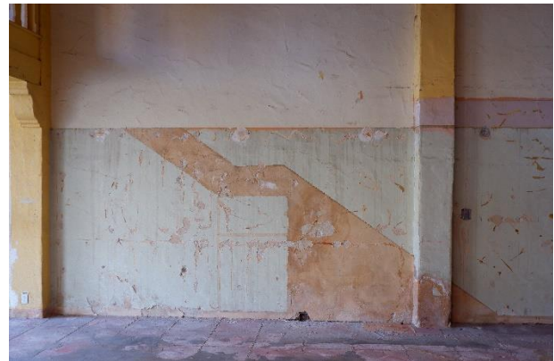
Figure 7. Ghost mark from original stair to mezzanine along the southeast wall, December 7, 2021.
