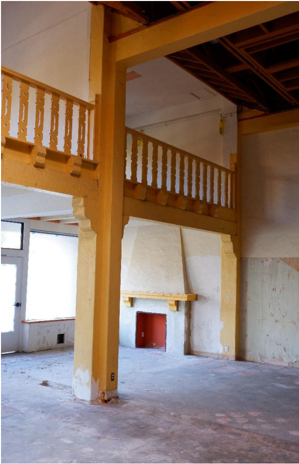
Figure 5. Interior mezzanine with adzed wood beams, posts, and joints, and decorative railing, December 7, 2021.
