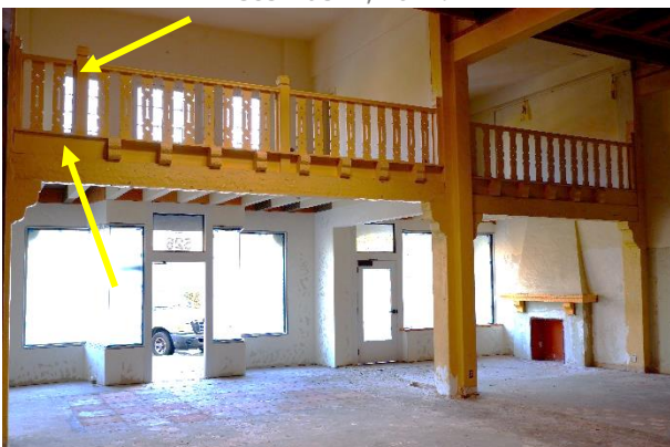
Figure 8. Front mezzanine, December 7, 2021. The location of the original stair to the central mezzanine area is visible by missing adzed brackets and extra newel post, indicated by yellow arrow.
