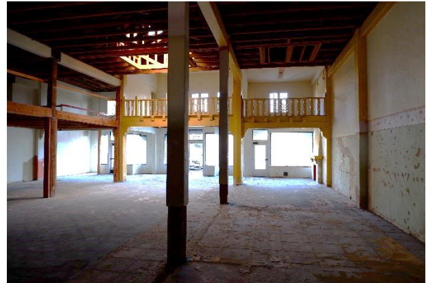
Figure 6. Original front mezzanine (right) and non-original mezzanine (left) along the northwest wall, December 7, 2021.
