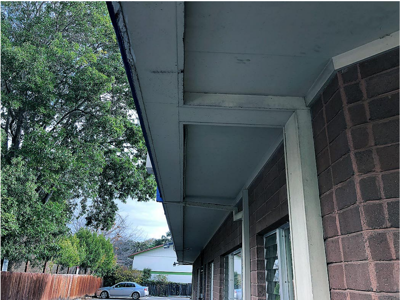
TYPICAL CANTILEVER SOFFIT
