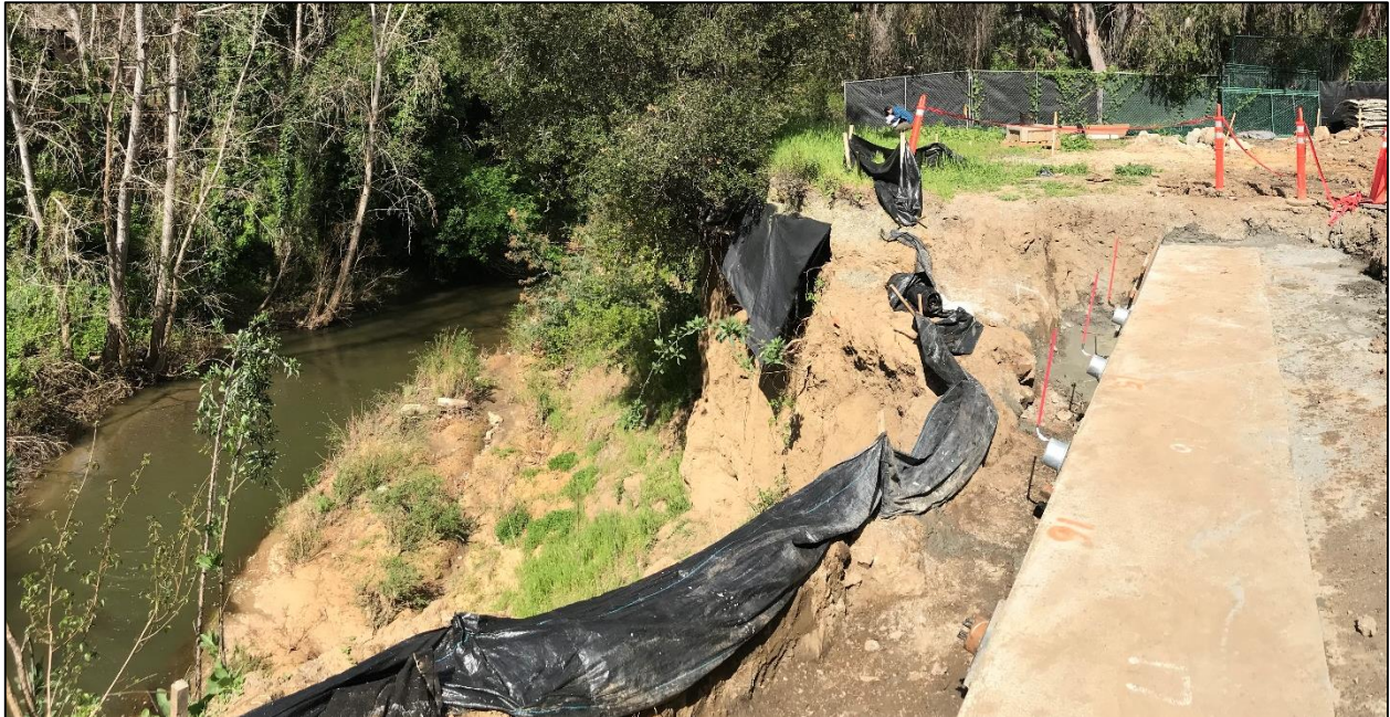
Photograph 3. View looking northwest along top of bank of creek. Photo depicts installation of concrete shear pin wall and set back from the top of bank. Cribwall work would occur along the lower sections of bank depicted here. Photograph taken March 21, 2019.
