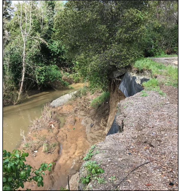
Photograph 6. Photograph looking downstream depicting acceleration of bank failure during 2016-2017 rainy season. Photograph taken March 23, 2017.
