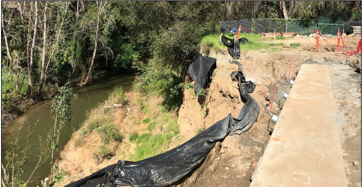
Photograph 3. View looking downstream, northwest, along top of bank of creek. Photograph depicts installation of Phase I concrete shear pin wall set back from the top of bank. Photograph taken March 21, 2019.
