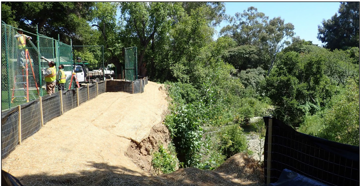
Photograph 4. View looking upstream, southeast, along top of bank of the creek within the Project Area. Photograph depicts completed Phase I shear pin wall construction. Photograph taken May 13, 2019.
