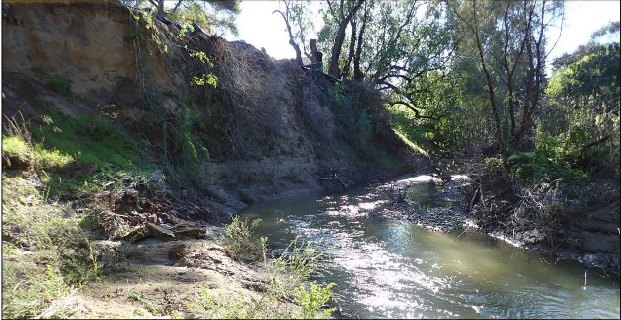
Photograph 1. Photograph looking upstream at the approximately 30-foot tall near vertical bank failure along San Francisquito Creek. Evidence of slumped debris and matted or destroyed vegetation can be seen on the east bank. The crib wall will be installed along the east bank to protect against future erosion and provide long-term stabilization. Photograph taken February 22, 2019.
