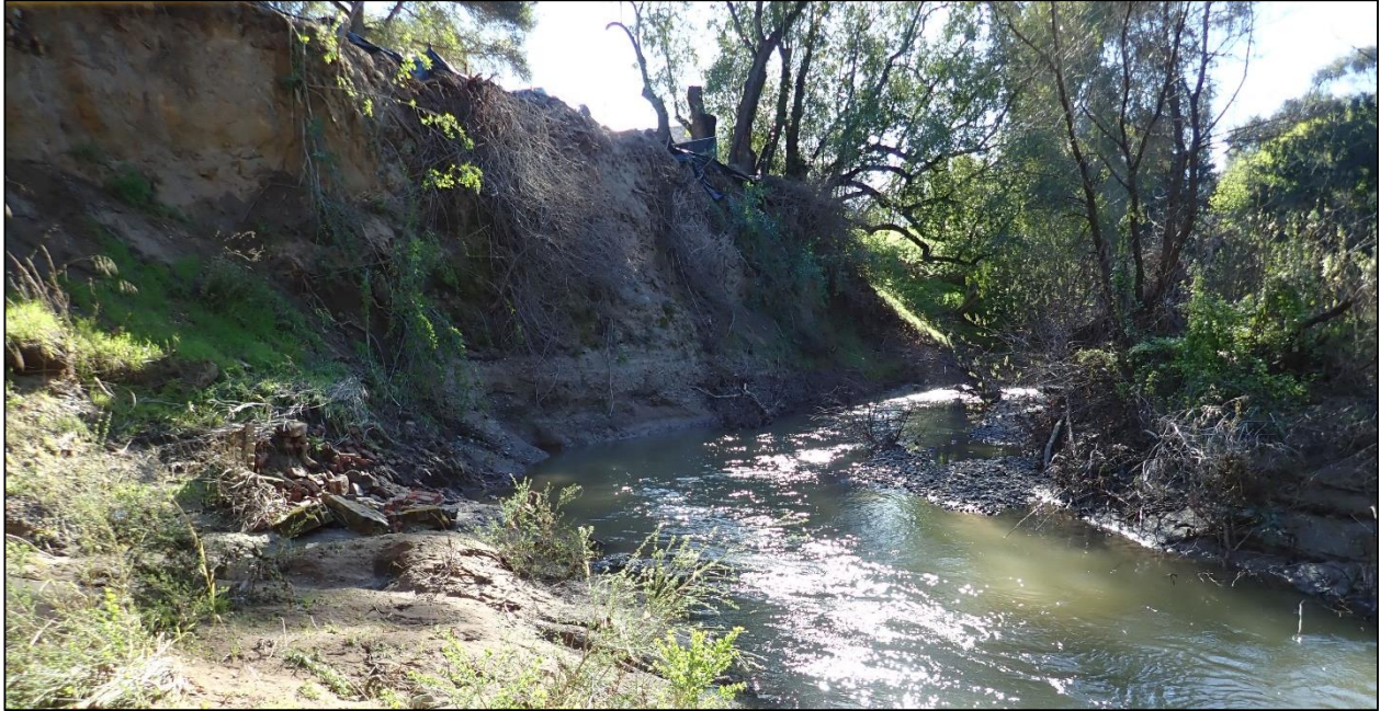
Photograph 1. Photo depicts the approximately 30-foot tall near vertical bank failure along San Francisquito Creek. Evidence of slumped debris and matted or destroyed vegetation can be seen on the east bank. The crib wall will be installed along the east bank to protect against future erosion and provide long-term stabilization. Photograph taken February 22, 2019.
