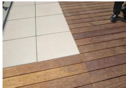
Unit Paving on Pedestals and Wood Deck
