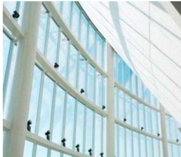
7 KAWNEER 1600 SS CURTAIN WALL SYSTEM WITH CONCEALED MULLIONS
