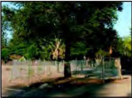
IMAGE 2.15-2 Tree Protection Fence at the Dripline
