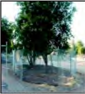
IMAGE 2.15-1 Tree Protection Fence at the Dripline
