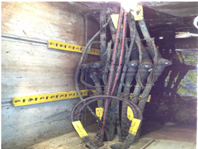
Electric underground cable vault
