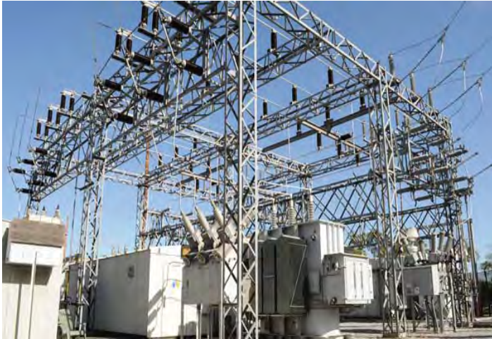
Electric Substation transformer and bus structure
