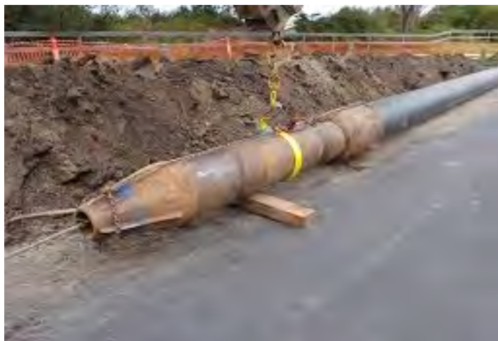
Sewer Main Replacement Project using Pipe Bursting Method
