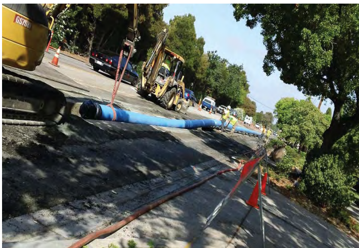
16" HDPE pipe ready to be installed by open trench method
