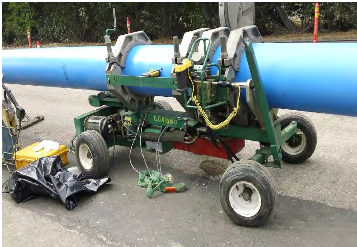
16" HDPE pipe being fused prior to installation
