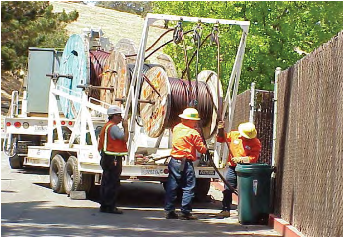
Electric crews installing new underground cables
