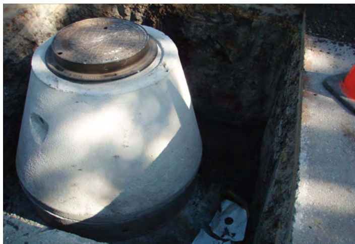
Sewer manhole base
