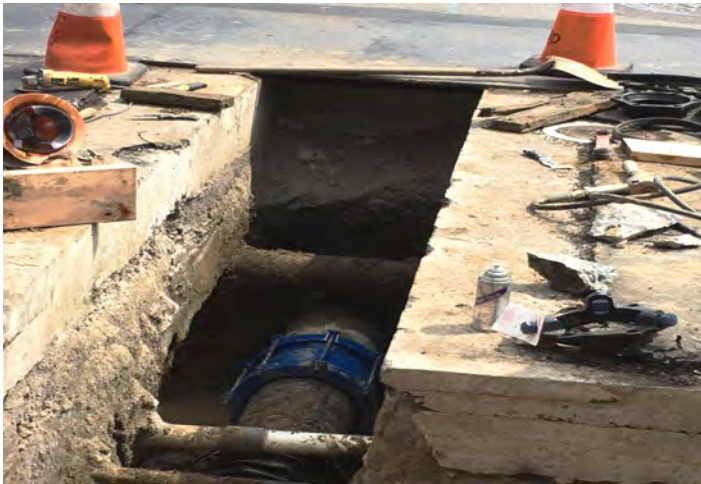
Installed 16" HDPE pipe waiting to be backfilled
