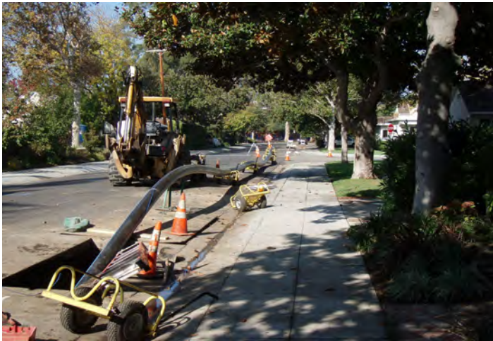
Installation of 8" HDPE pipe by directional drilling method
