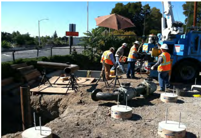
Installation of new HDPE gas service main
