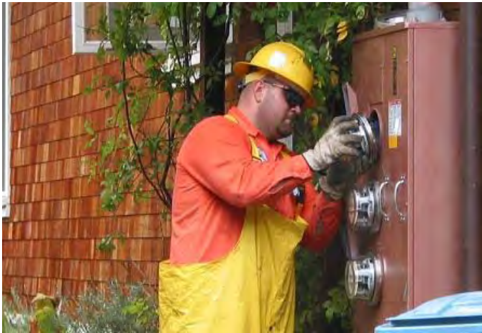
Electric Troubleshooter installing an electric meter to provide service to a customer
