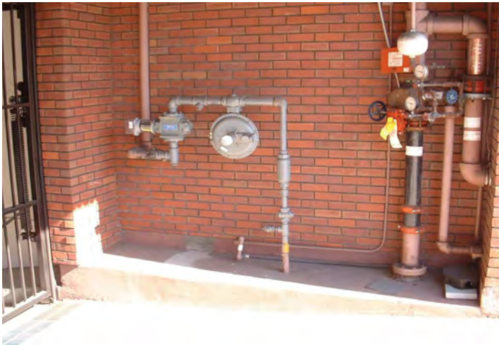
New gas service meter and regulating equipment
