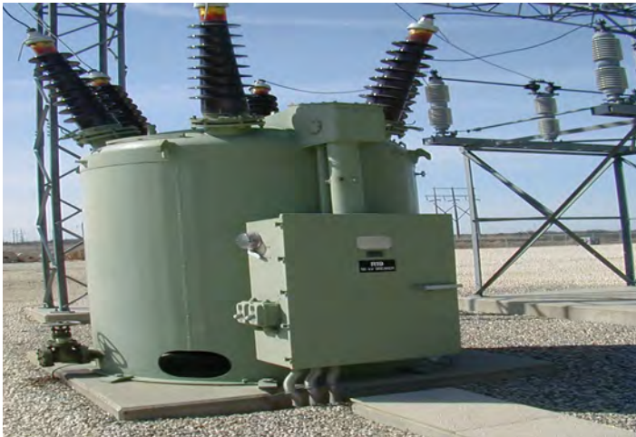
High voltage circuit breakers
