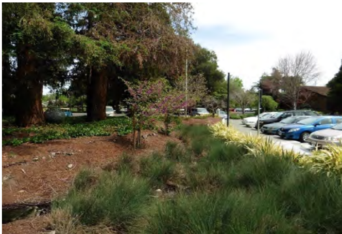
Bioretention measure at Rinconada Library that treats on-site stormwater runoff, 2014
