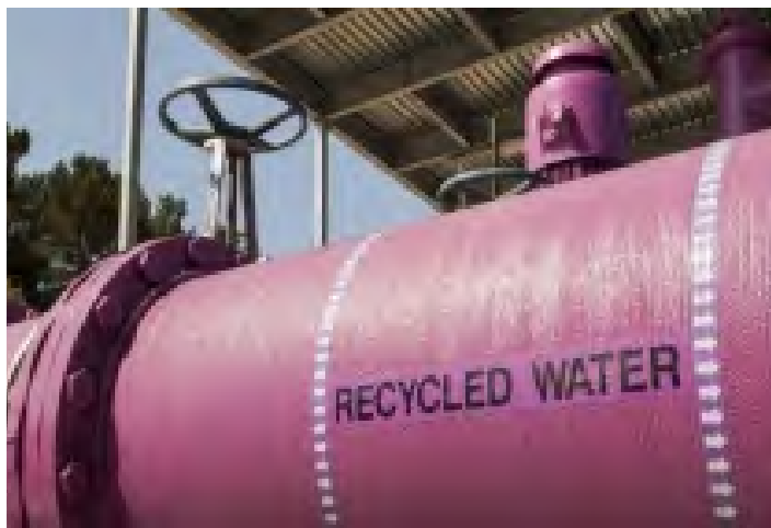
Recycled water piping
