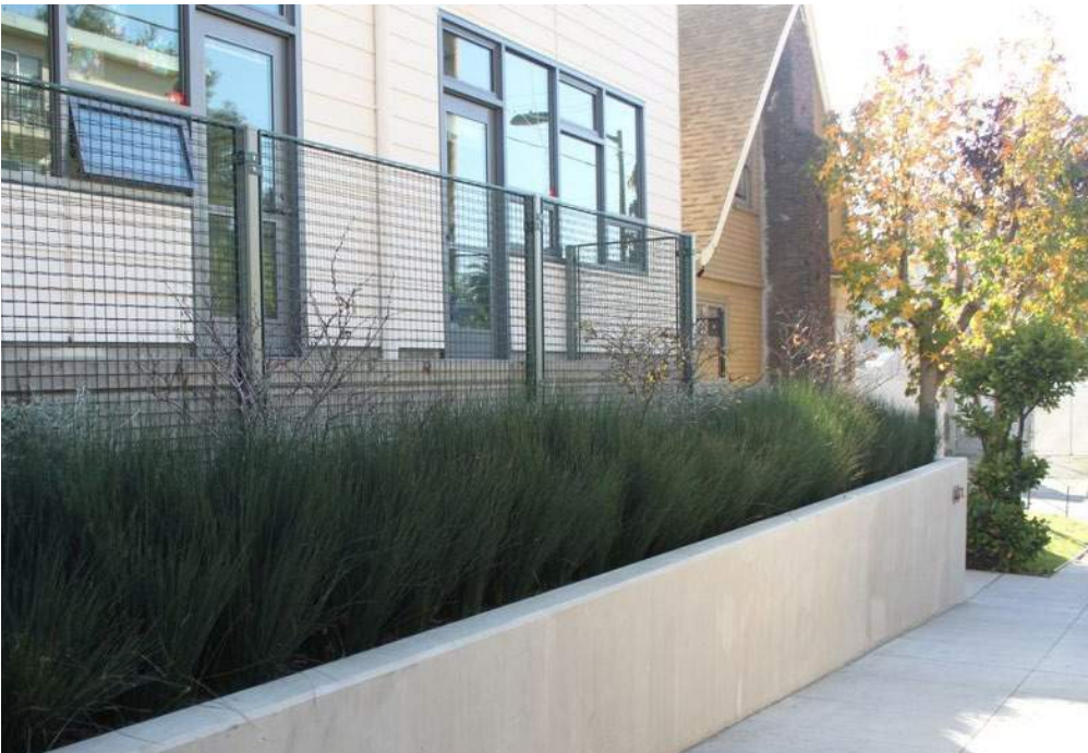
Raised Concrete Treatment Planter Height above grade varies in different site conditions. See plans
