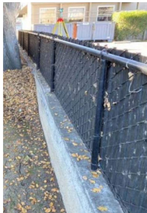
Existing Concrete Foundation Wall (Along Property Line Near Large Coast Live Oak) to Remain
