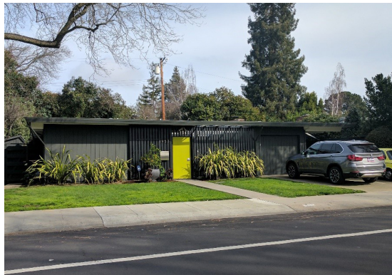
Top: Garage doors are solid and clad in vertical wood board, similar or identical to the wall cladding.
