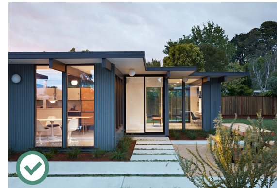
Two examples of successful one-story rear additions to existing Eichler homes. These examples add additional living space while preserving the valued indoor-outdoor connection of the rear yard and blend seamlessly with the original home. Source: Courtesy of Klopff Architecture. Copyright ©2017 Mariko Reed.
