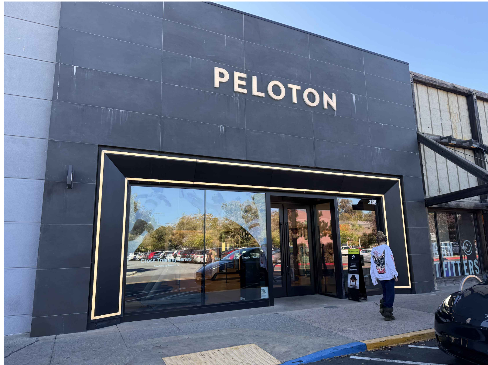
4 EXISTING DAYTIME PHOTO
