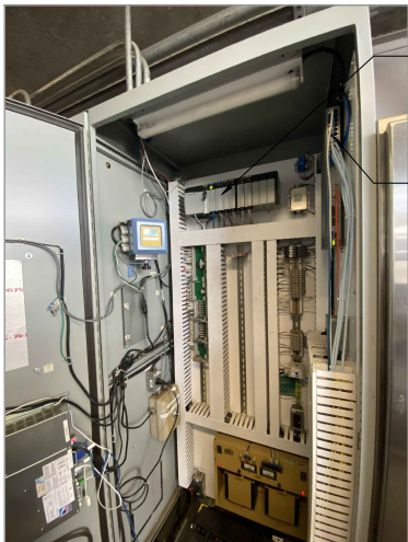
EXISTING PLC PANEL MCP-1 PHOTO
