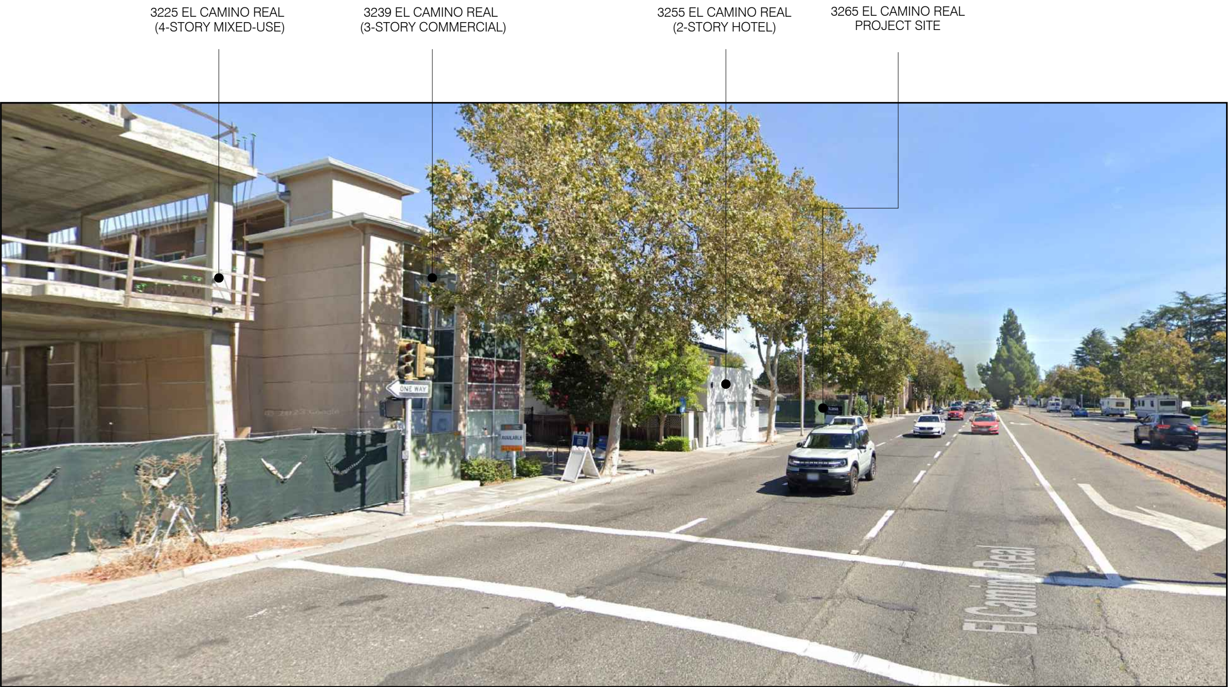
3 VIEW FROM EL CAMINO REAL - LOOKING SOUTHEAST
