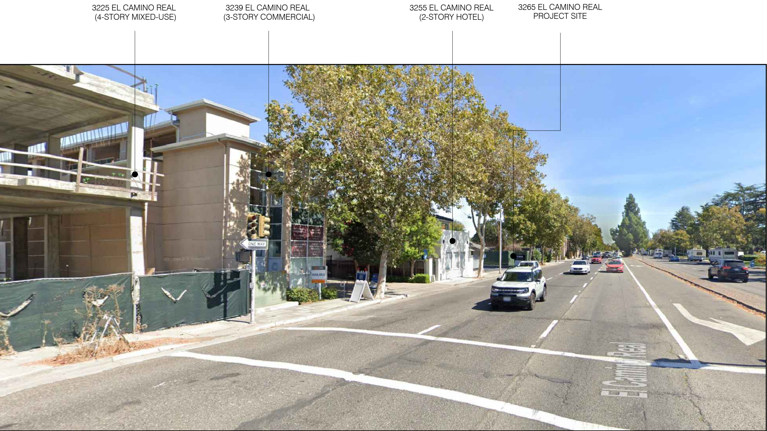
3 VIEW FROM EL CAMINO REAL - LOOKING SOUTHEAST
