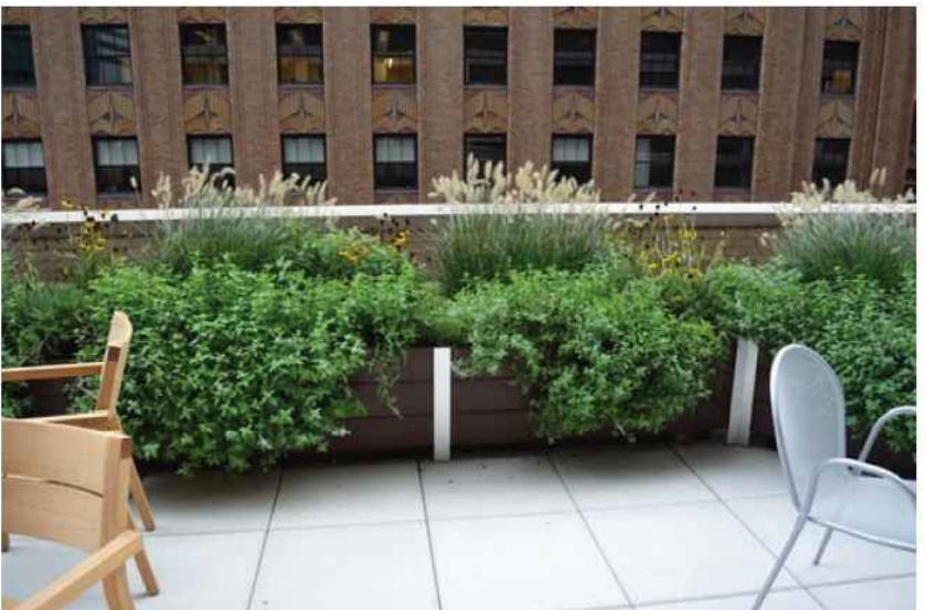
Vegetation prevents people to come close to parapet
