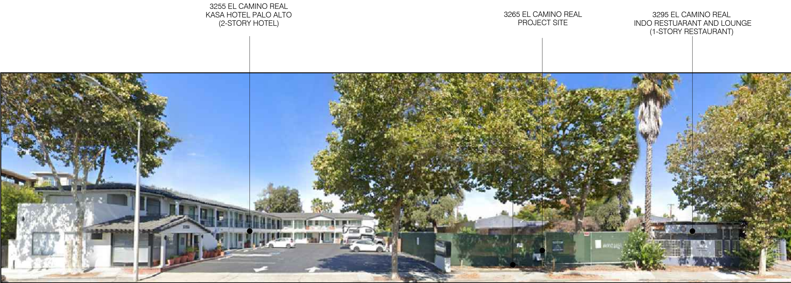
2 VIEW FROM EL CAMINO REAL - LOOKING AT FRONT OF SITE
