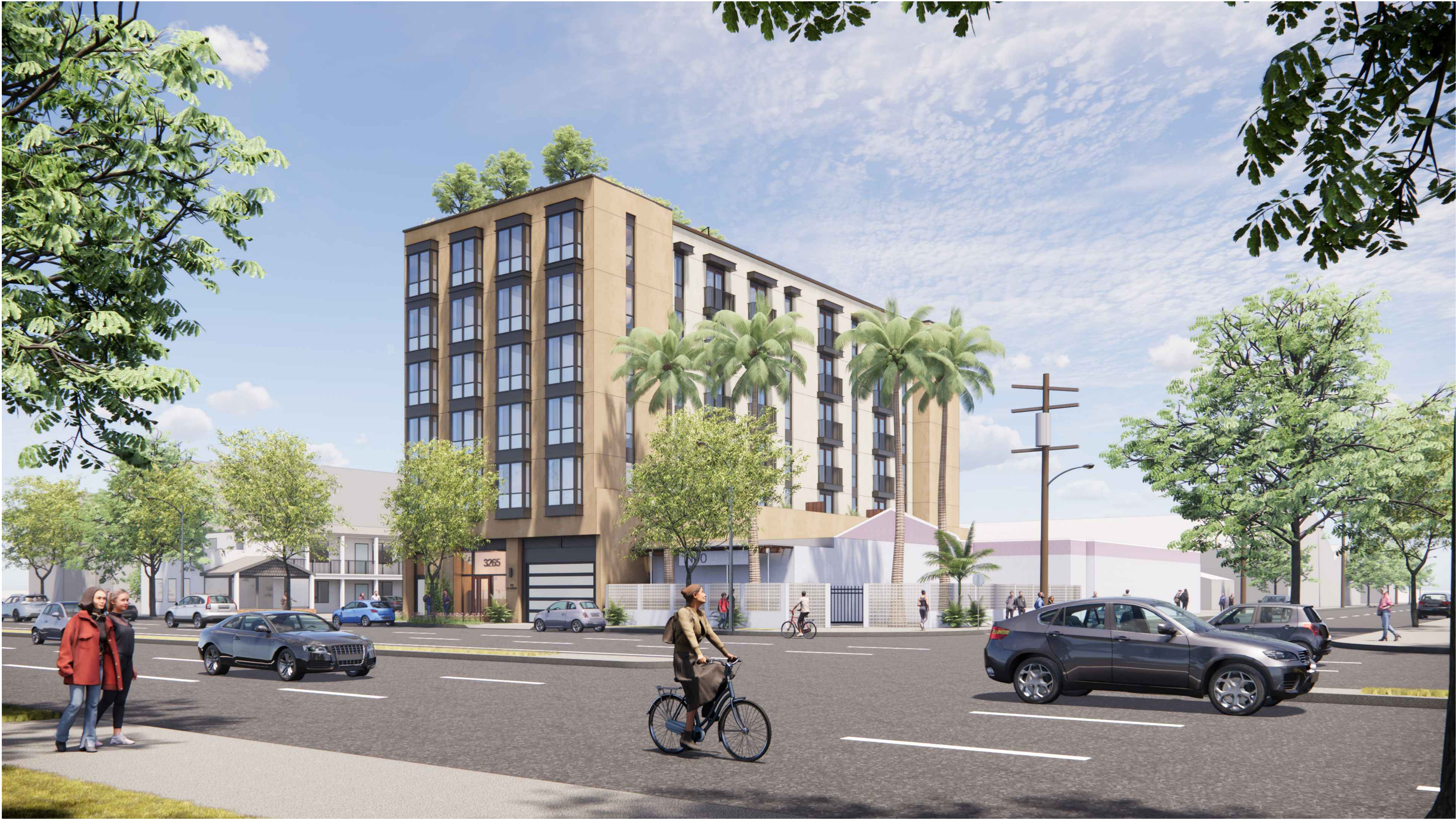
1 - VIEW LOOKING FROM SOUTHEAST
