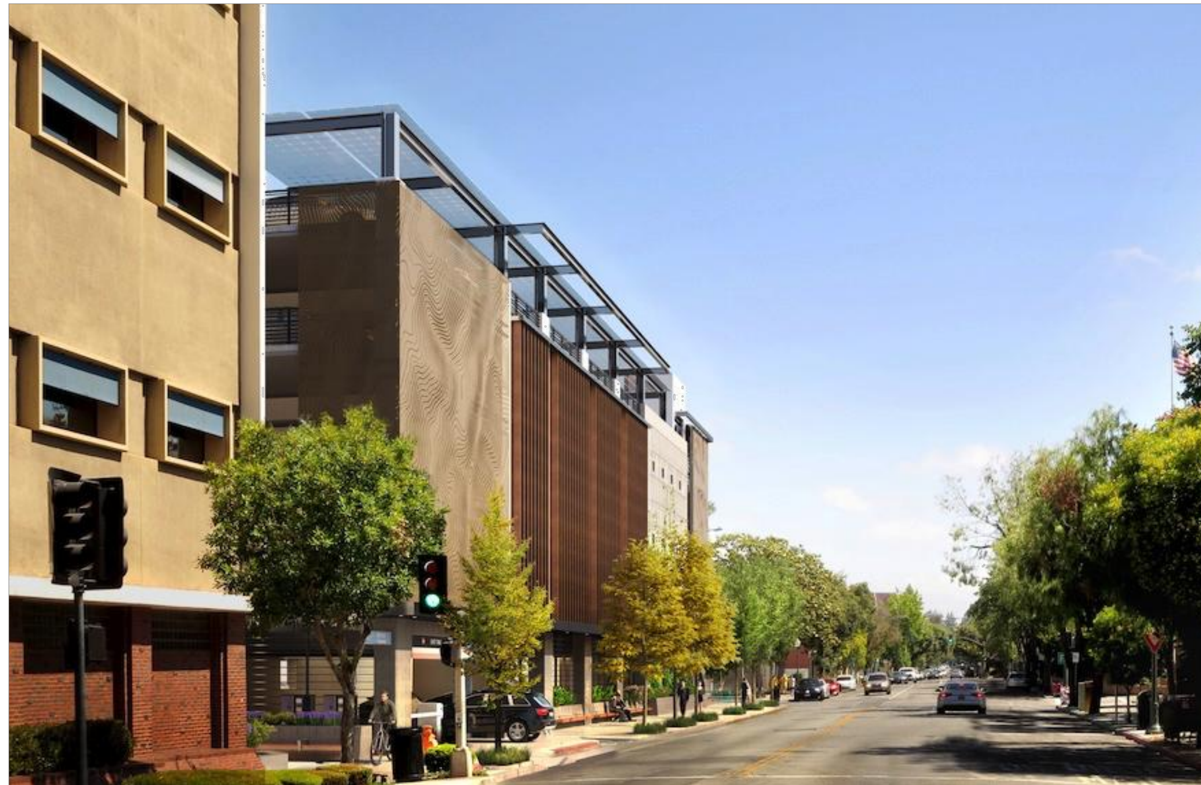
HAMILTON AVENUE, VIEW, LOOKING NORTH-EAST TO WAVERLEY
