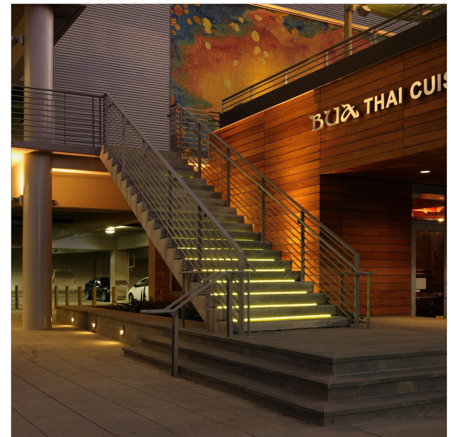
CLAREMONT MUNICIPAL PARKING GARAGE FEATURE STAIRS AND RAILINGS
