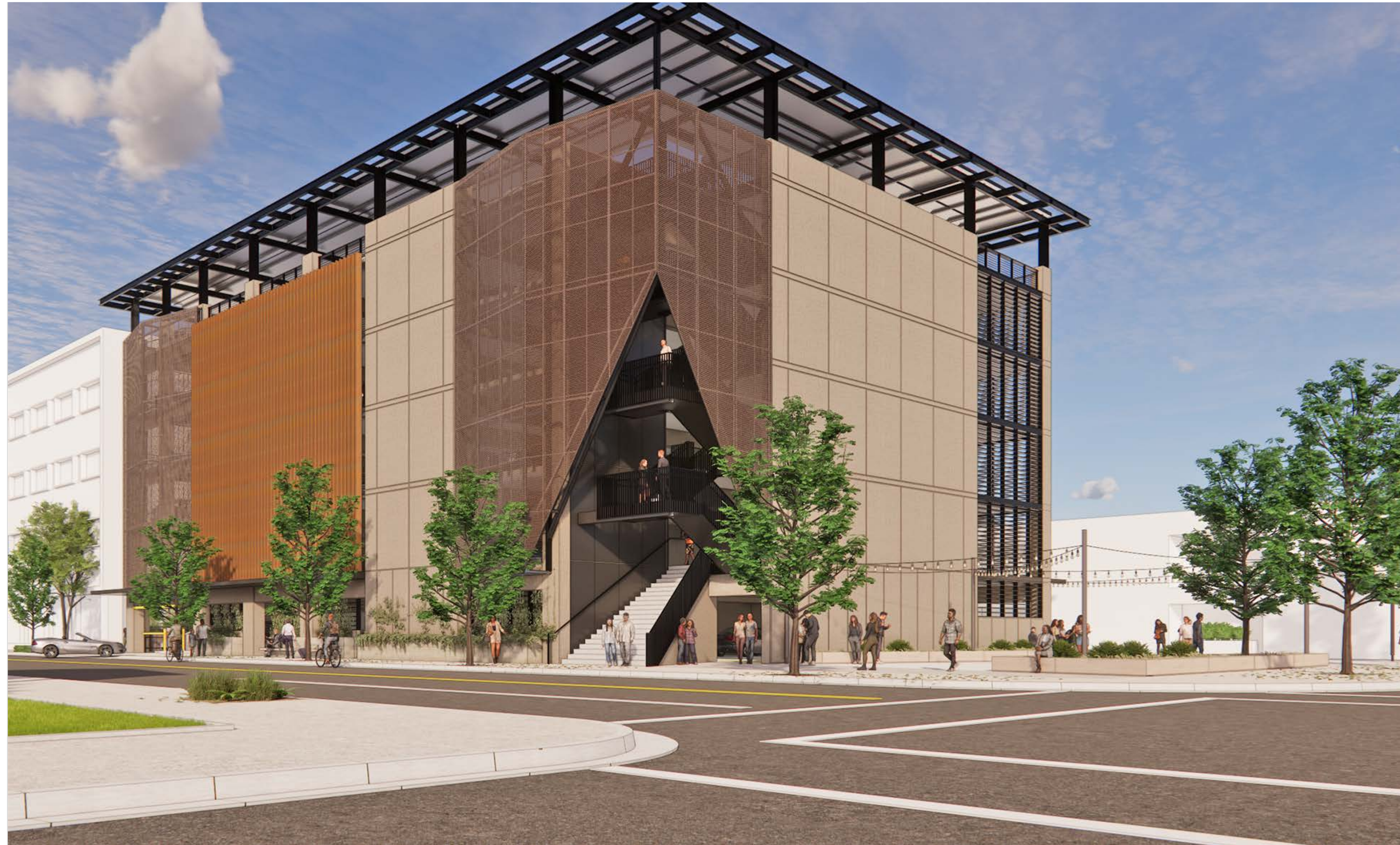
VIEW OF GARAGE FROM CORNER OF HAMILTON AVE. AND WAVERLEY ST.
