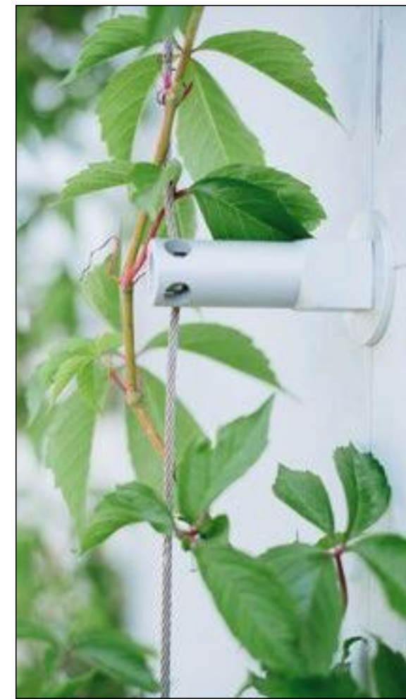
STAINLESS STEEL CABLE SYSTEM TO SUPPORT CLIMBING VINES
