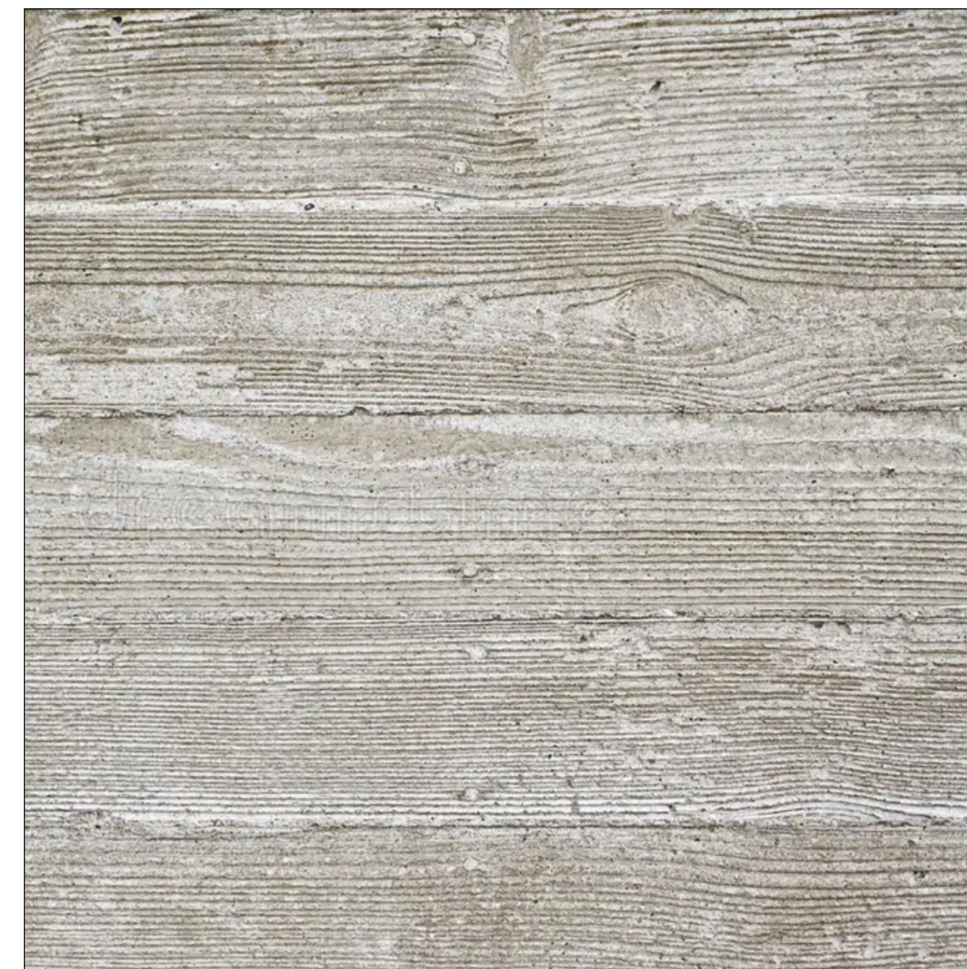
BOARD FORM CONCRETE, NATURAL COLOR
