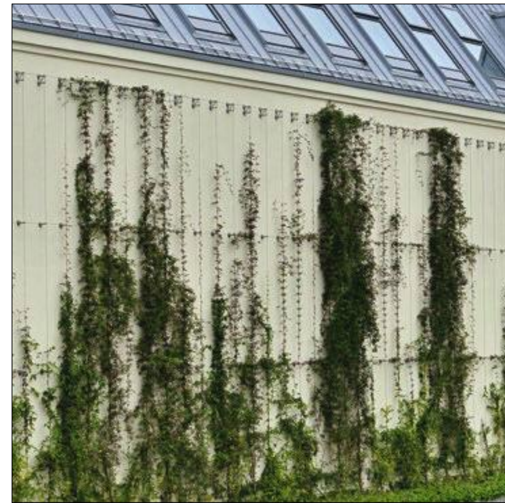
STAINLESS STEEL CABLE SYSTEM TO SUPPORT CLIMBING VINES
