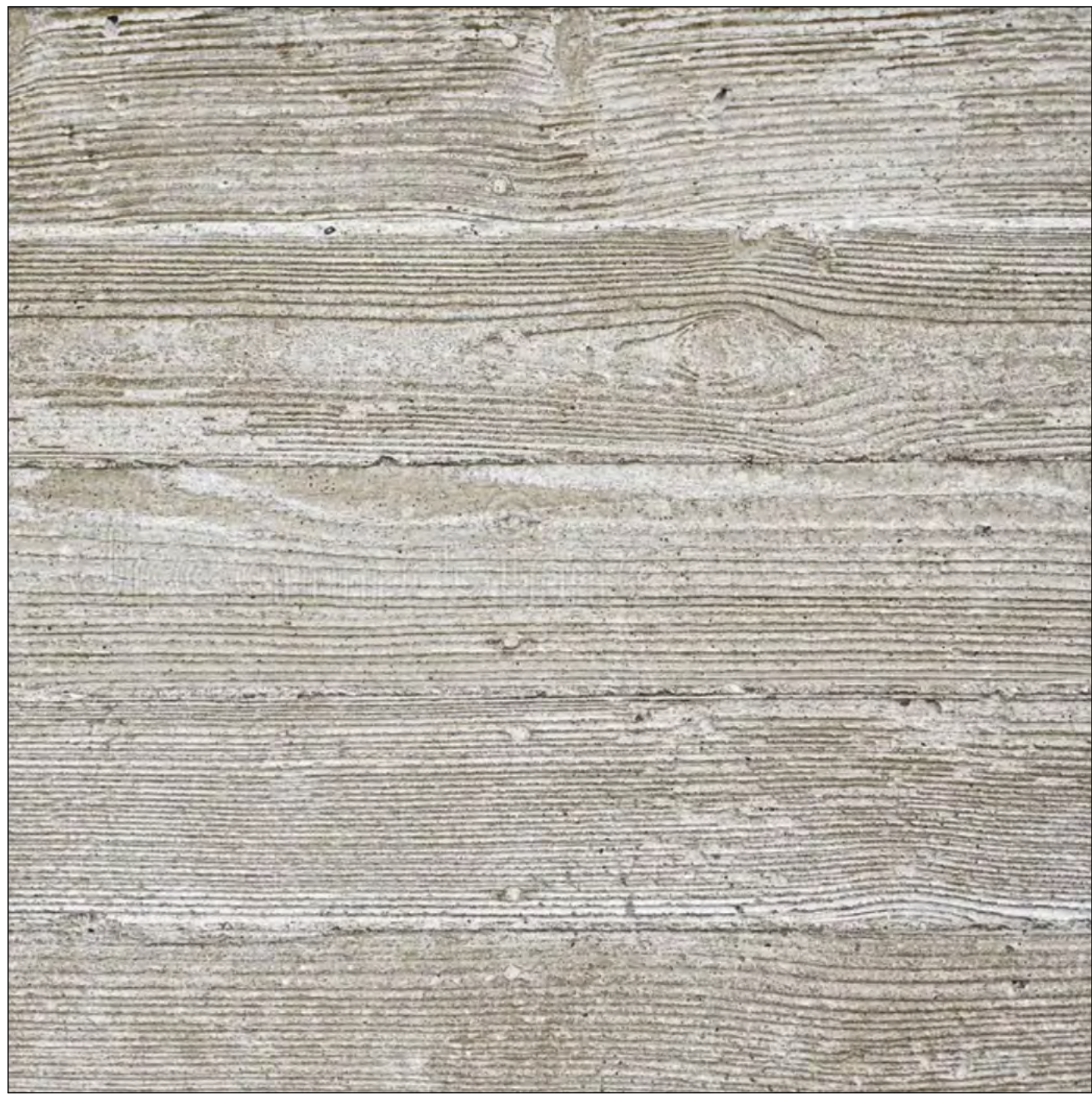
BOARD FORM CONCRETE
