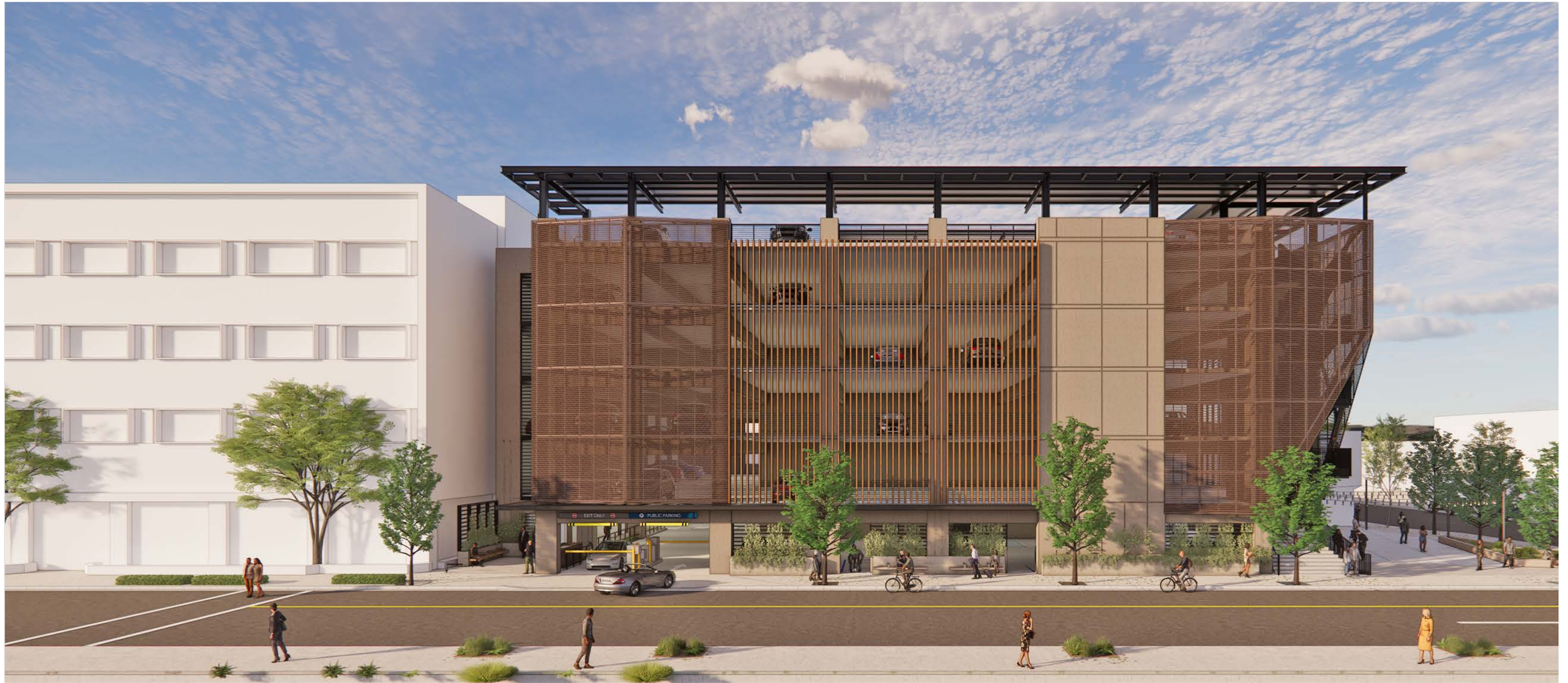
VIEW OF GARAGE AT HAMILTON AVENUE
