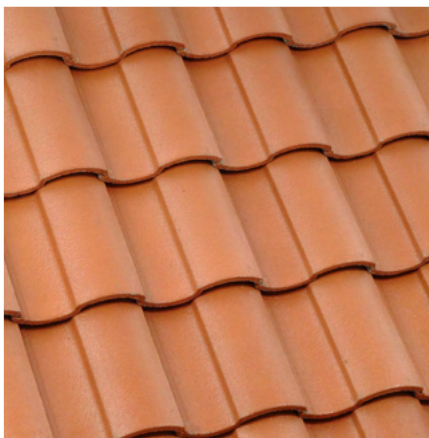
CLAY TILE ROOF 7
