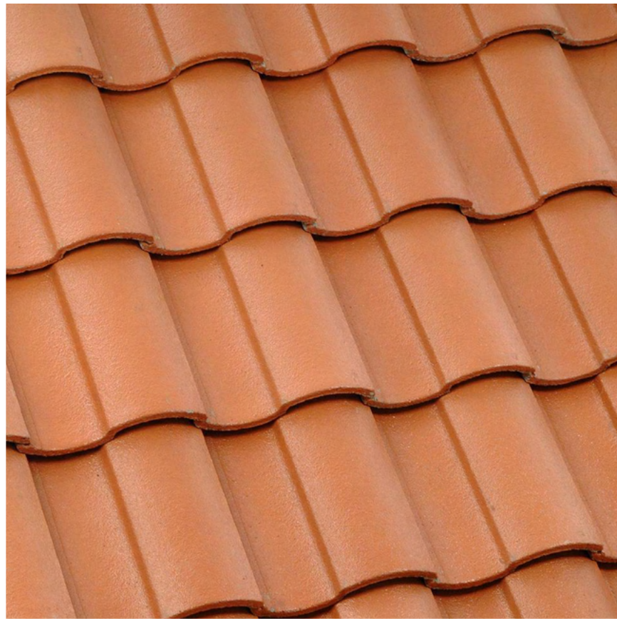
CLAY TILE ROOF
