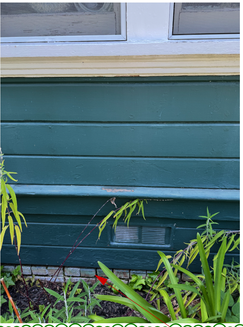
16 REMOVE (E) UNREINFORCED MASONRY FOUNDATION AND REPLACE W/ (N) CONCRETE FOUNDATION IN ACCORDANCE W/ PAMC CHAPTER 16.42 SEISMIC REHABILITATION REQUIREMENTS
