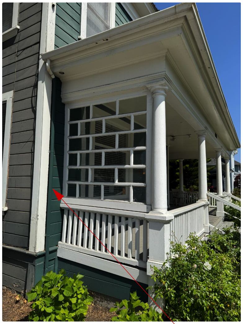
2 REPLACE ALL DOWNSPOUTS TO PORCH, TYP.
