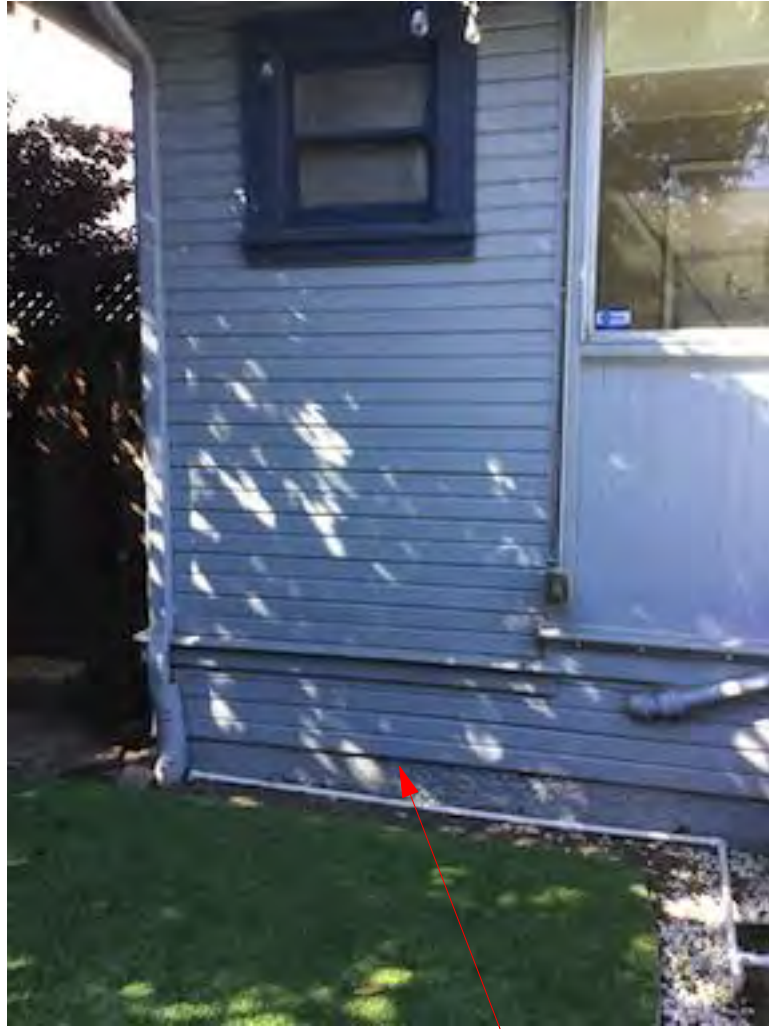
11A PATCH AND SACK EXPOSED CONCRETE FOUNDATION
