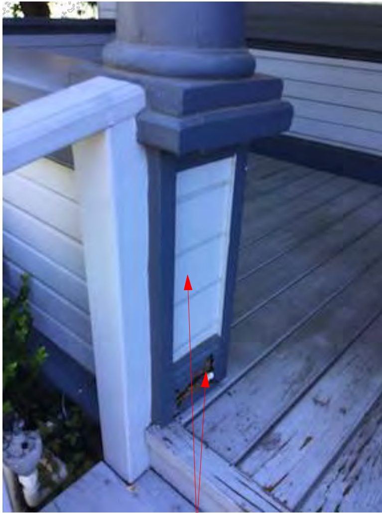
2A REPAIR /REMOVE/ REPLACE DAMAGED AND/ OR UNORIGINAL SIDING, TRIM & DECKING
