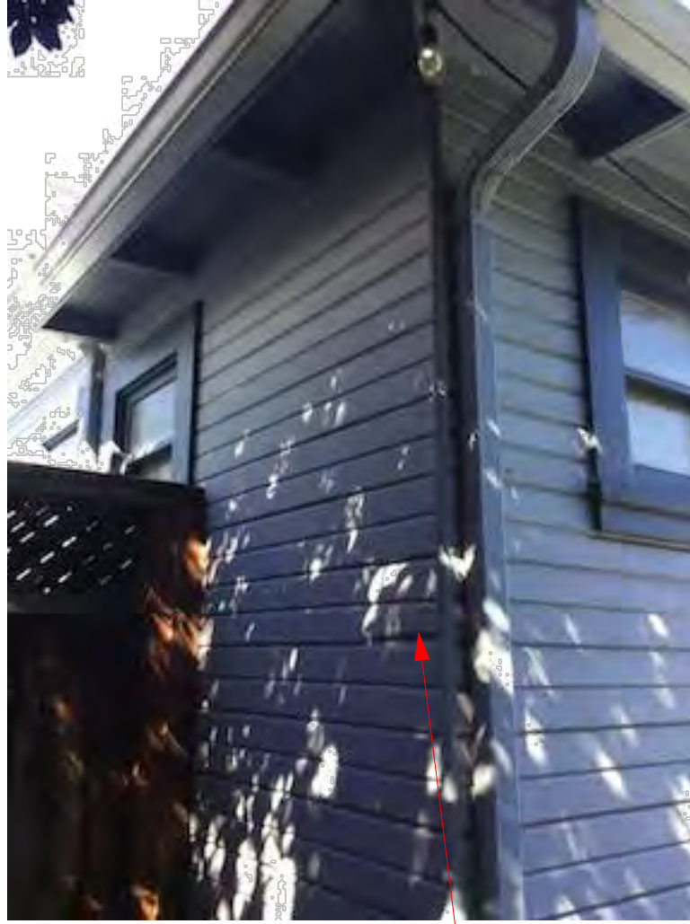
8 REPAIR /PATCH ANY DEFECTS IN ORIGINAL SIDING
