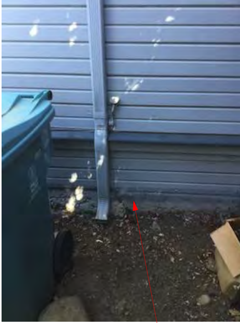
11B PATCH AND SACK EXPOSED CONCRETE FOUNDATION
