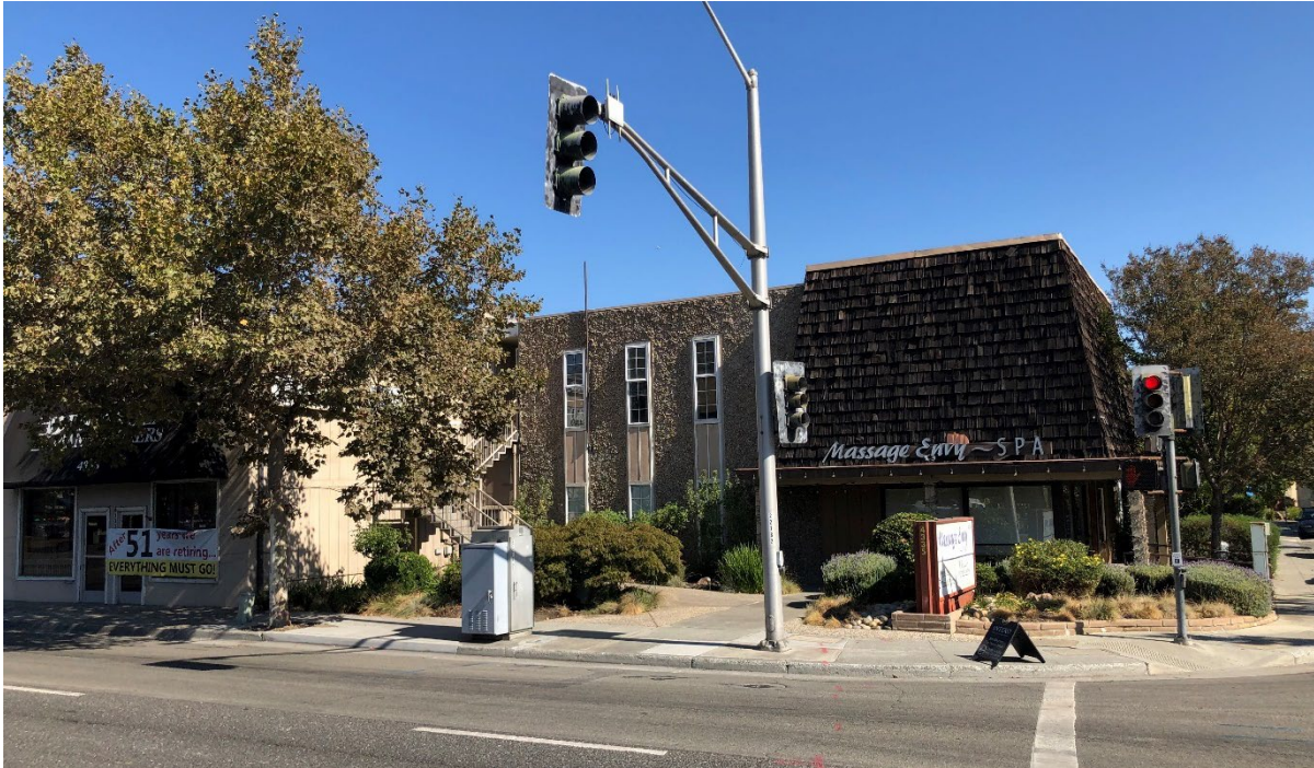
Photo 1: Buildings on the smaller (northern) parcel (APN 148-09-010), viewed looking northeast from El Camino Real.
