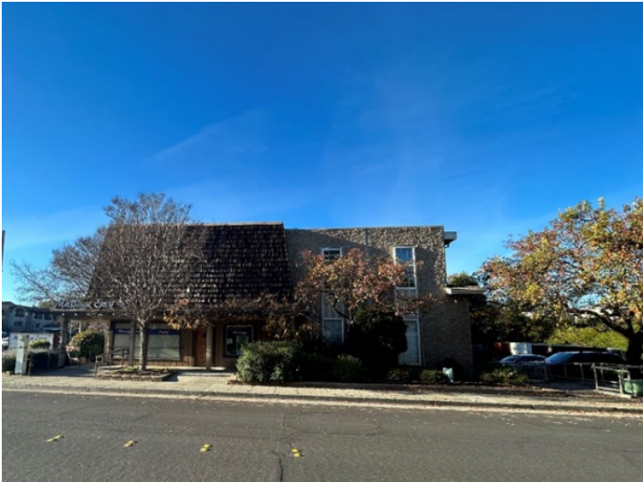
Photograph 2 4333-4335 E; Camino Real View: Front – South side Camera facing North Date: 1/2/2025
