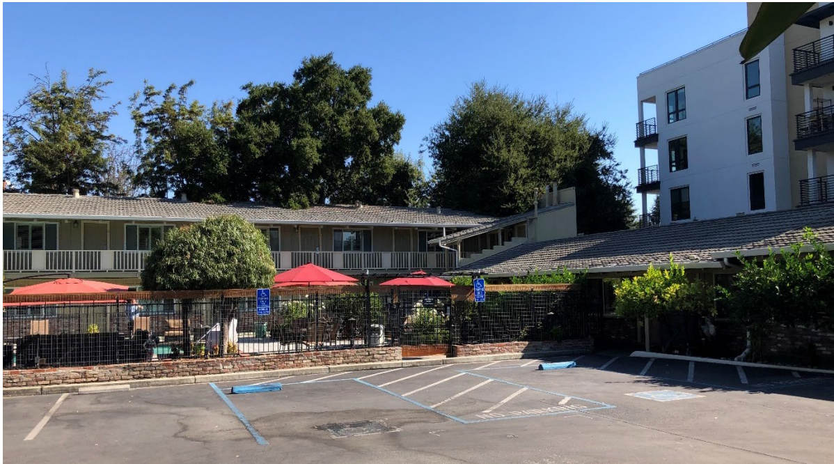
Photo 3: Existing building on the larger (southern) parcel (APN 148-09-011) and surface parking lot, viewed looking west from the interior of the site.
