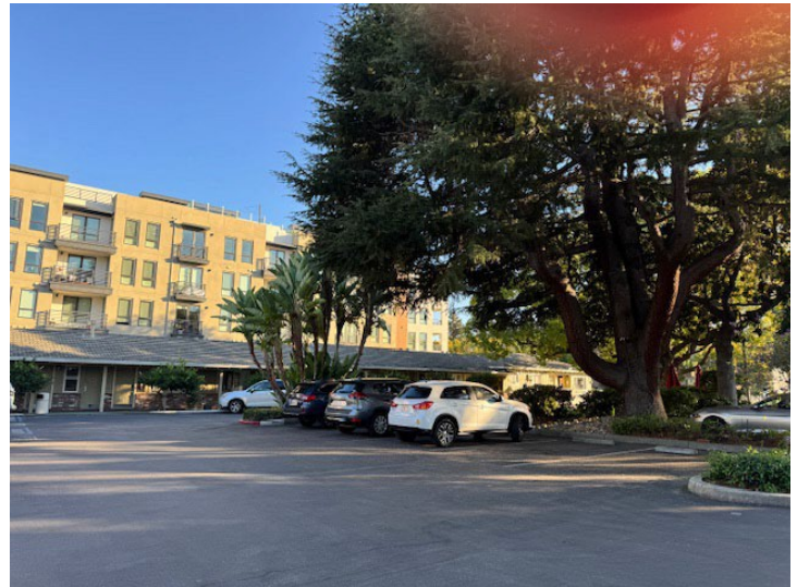
View looking at the center parking and landscaped area.
