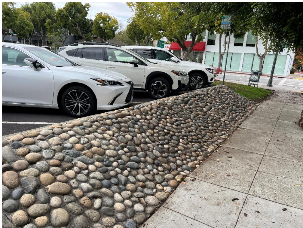
Photo 8: Subject Property northeastern border and berm (facing NW).
