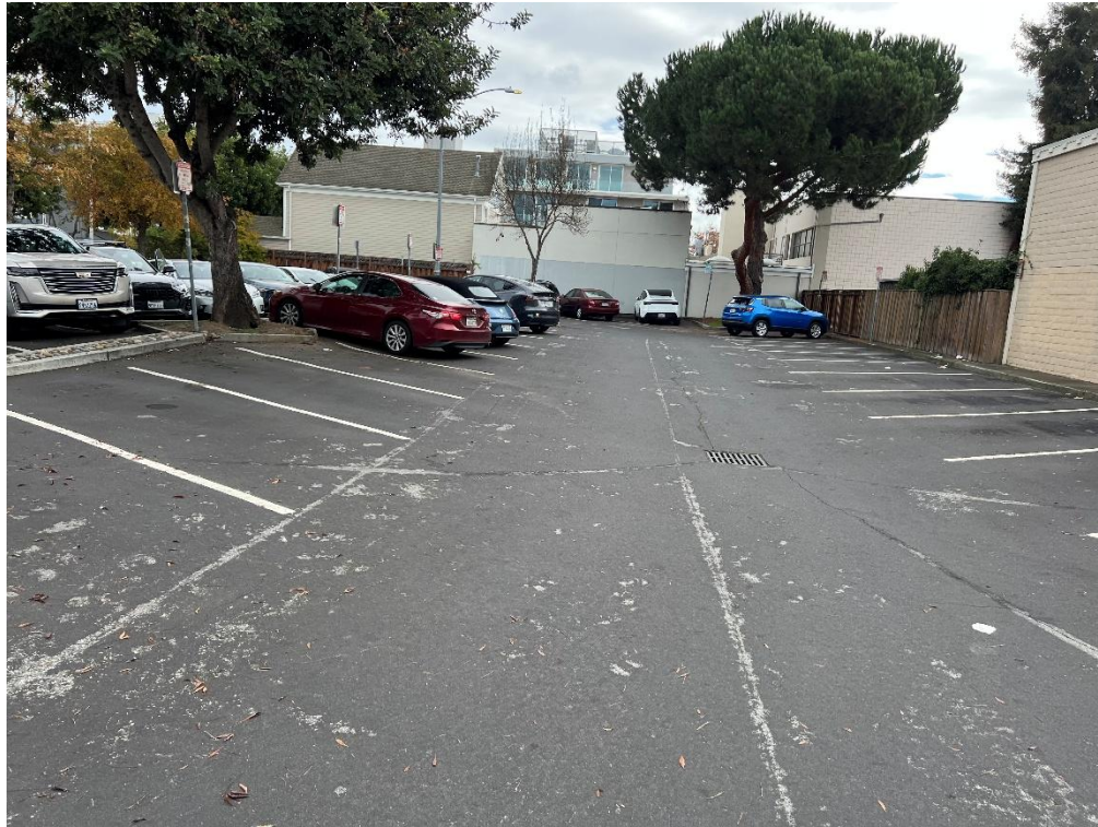
Photo 3: Subject Property and storm drain (facing SE).
