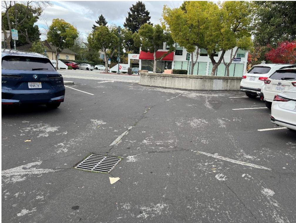
Photo 7: Subject Property and third storm drain (facing NW).
