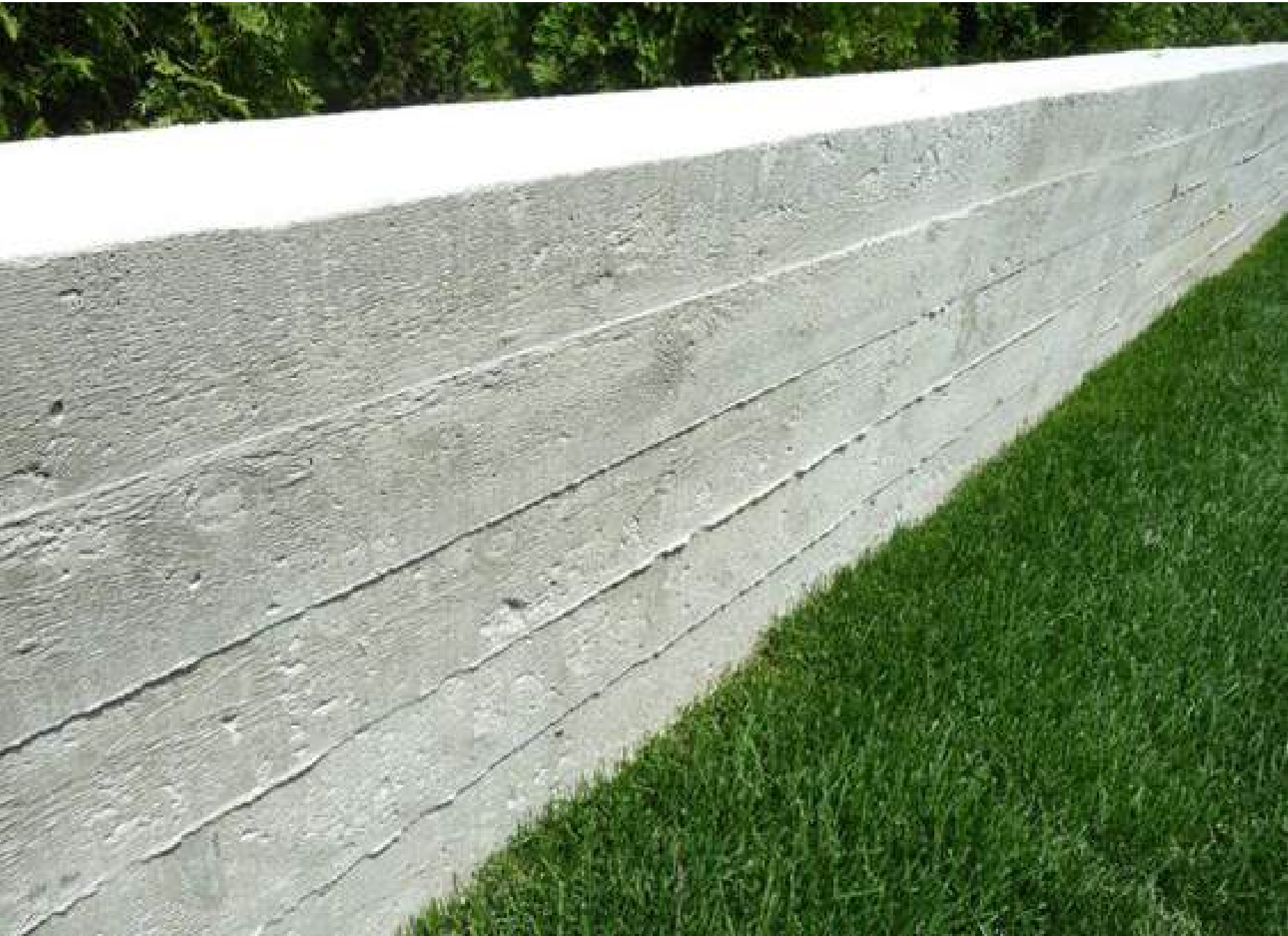
E - RETAINING WALLS - BOARD FORMED CONCRETE
