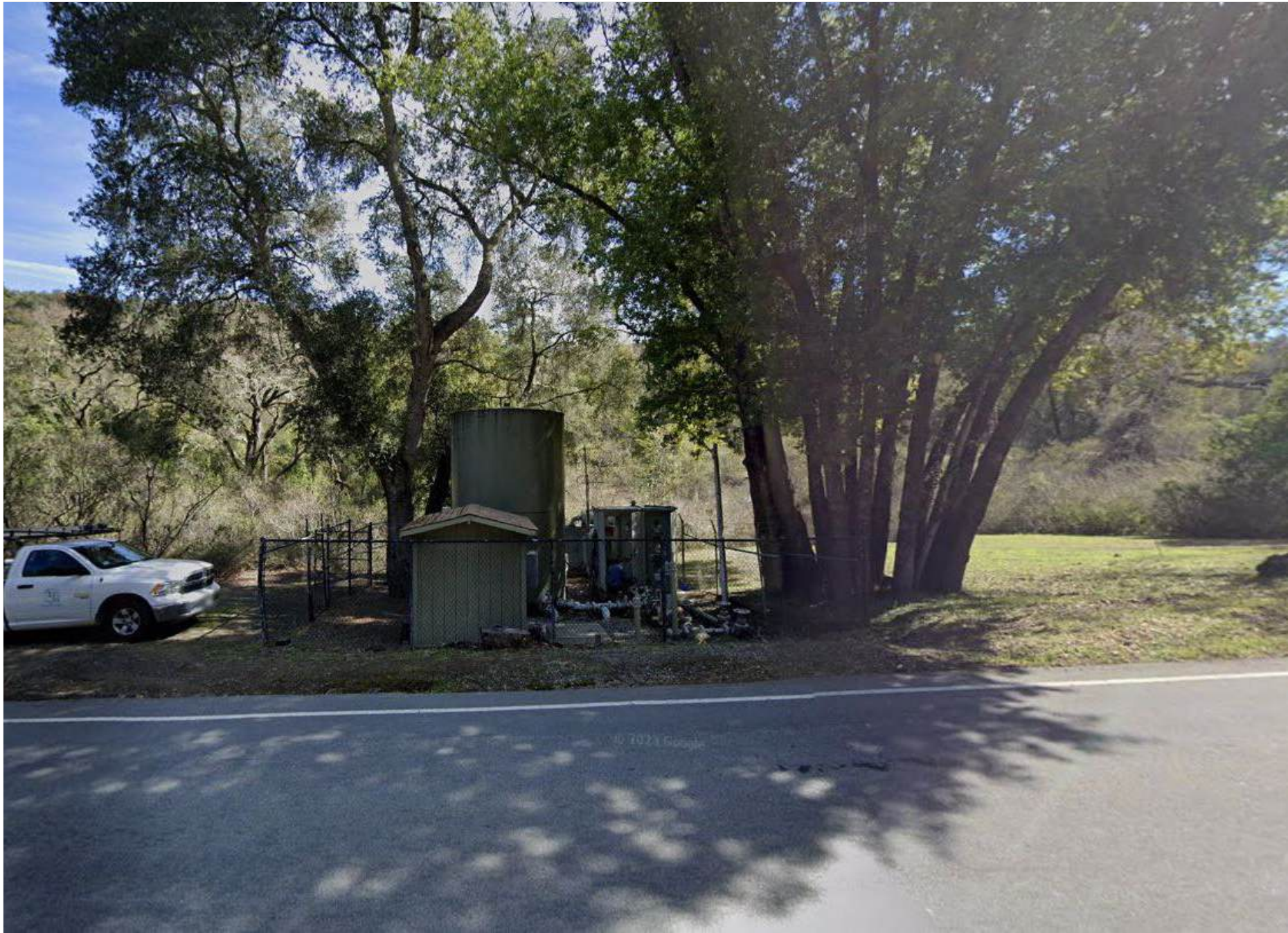
D - UTILITIES ENCLOSURE ALONG LOS TRANCOS RD.
