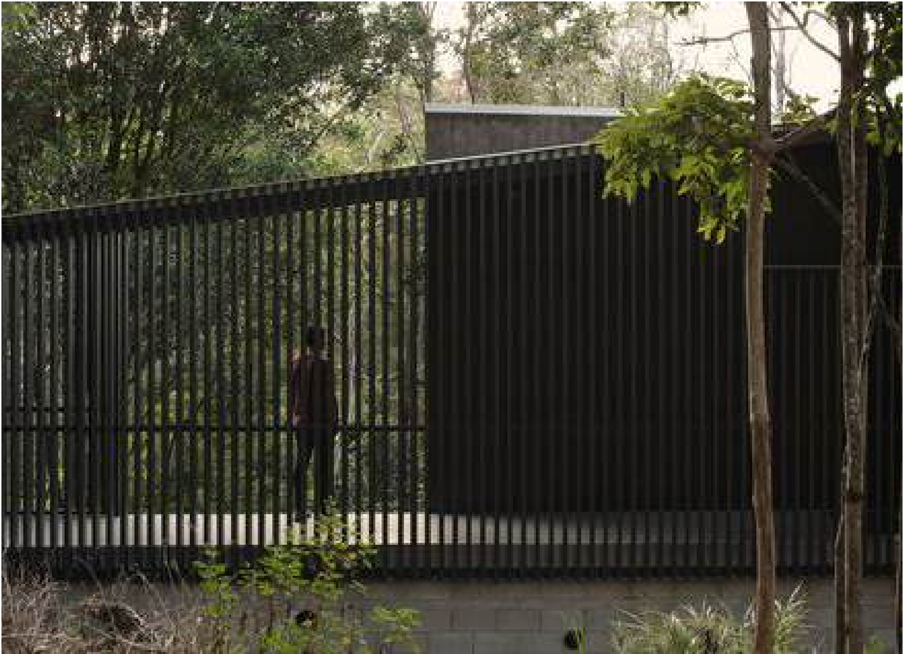
D - EXTERIOR SCREENING - FIXED METAL SLATS
