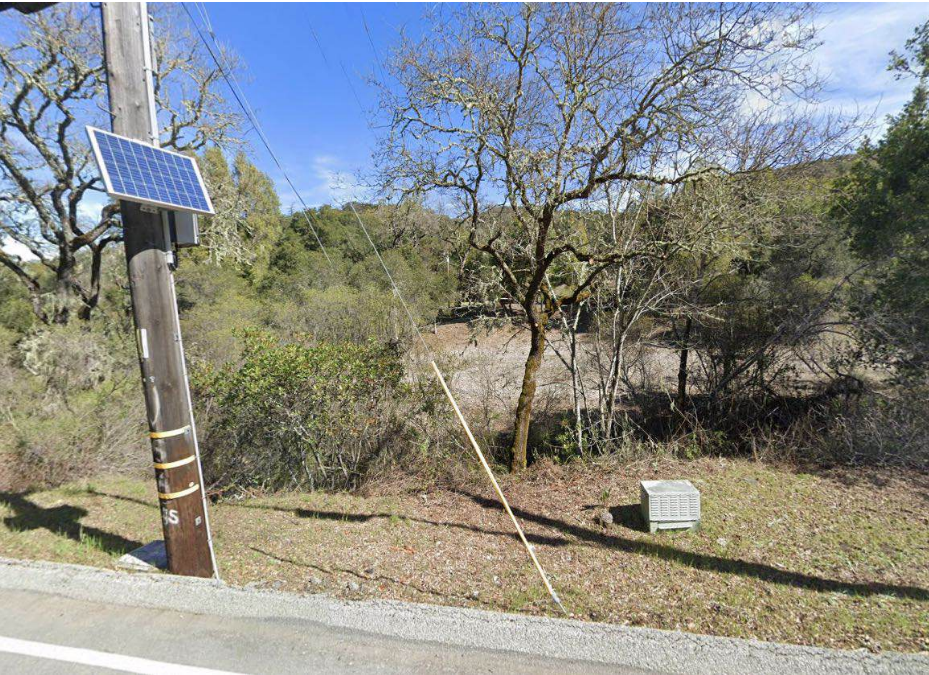
I - VIEW OF EXISTING UTILITY AT LOS TRANCOS RD.
