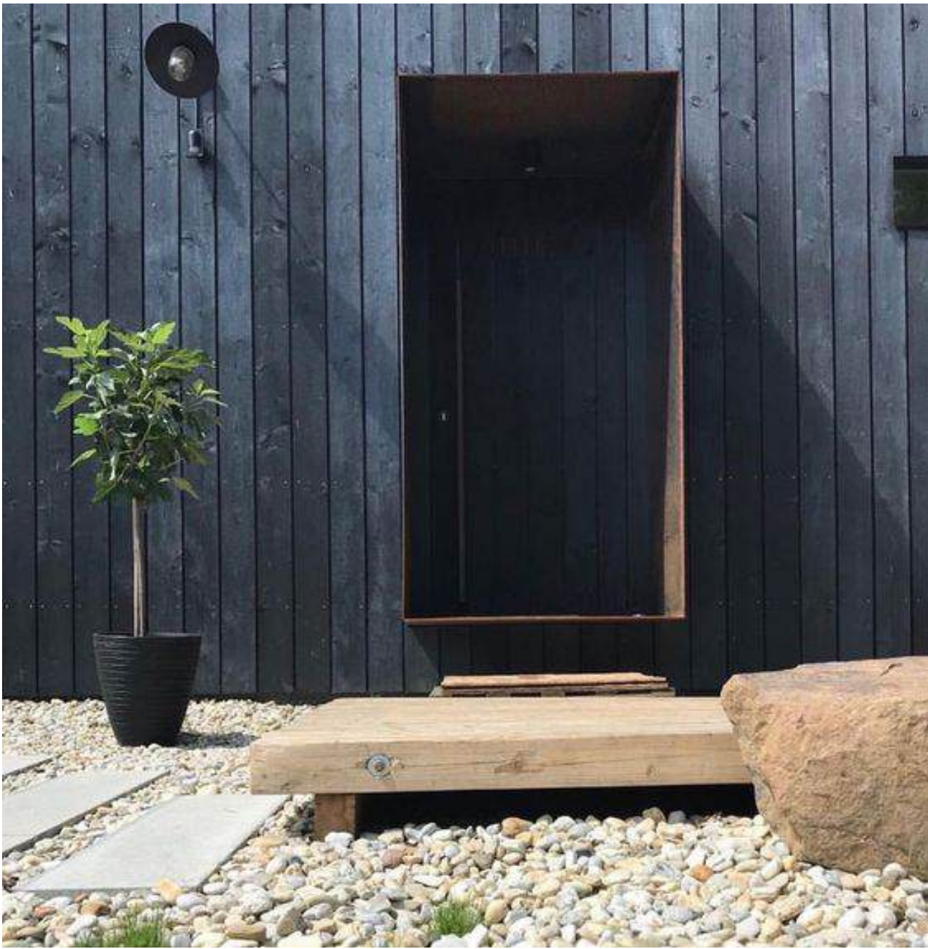
B - EXTERIOR CLADDING - SHOU-SUGI-BAN WOOD SIDING
