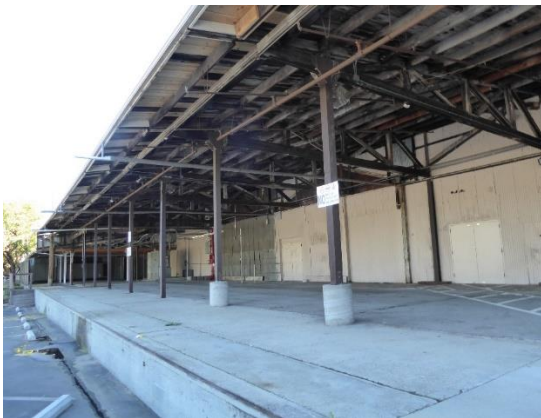
Figure 27. A portion of the concrete loading platform or cooling porch with its shed awning and wood post-and-beam supports in the middle section of the northwest façade. View northeast.
