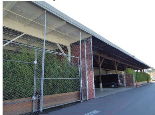
Figure 32. Wood post-and-beam construction under the awning at the south end of the northeast façade. View south.
