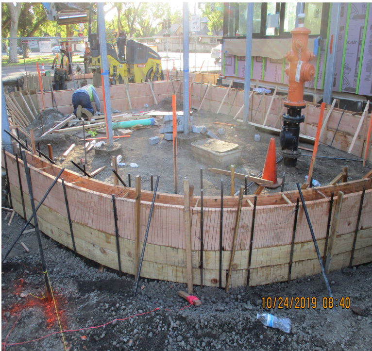
Curb and concrete flatwork installation at the north side of the fire station.
