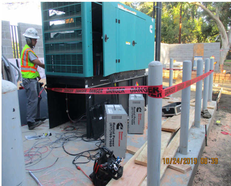
Emergency Generator testing and inspection.
