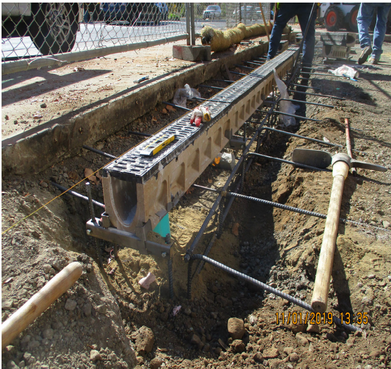
Trench drain installation at the main entry driveway at Embarcadero Road.
