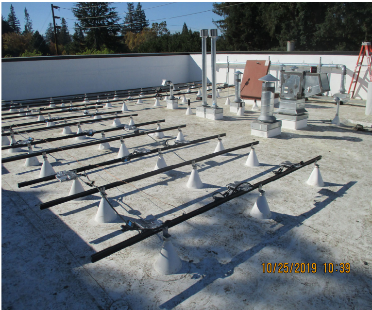
Solar panel roof-top mounting and horizontal supports.
