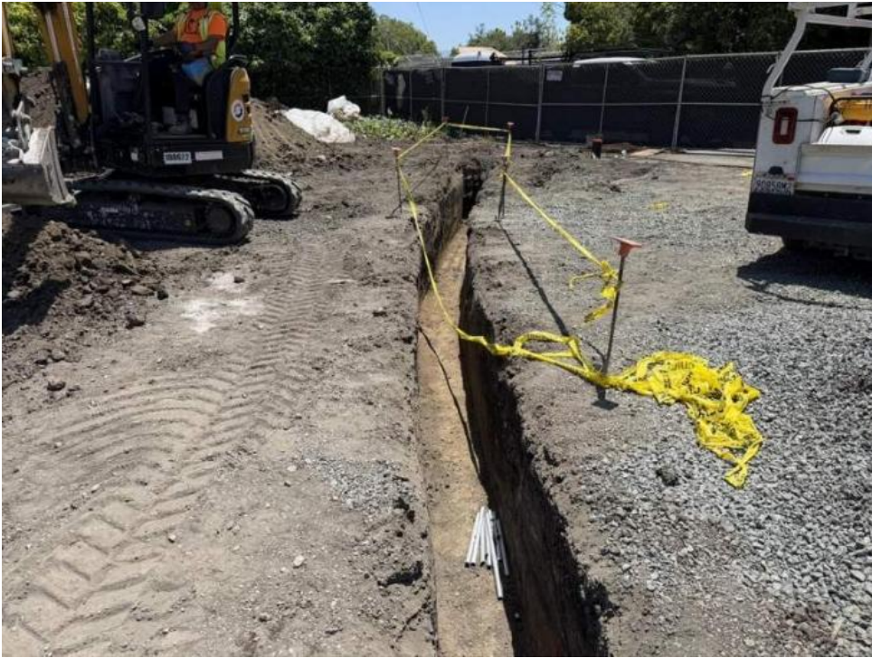
Trench and electrical conduits
