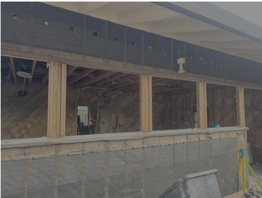
Exterior Window/Wall Demo
