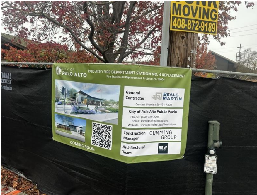
Site sign installed on site fence.
