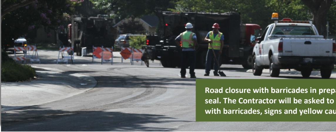
Road closure with barricades in preparation for the slurry seal. The Contractor will be asked to protect work areas with barricades, signs and yellow caution tape.
