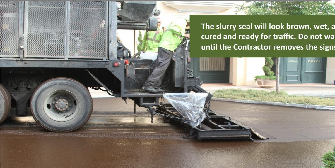
The slurry seal will look brown, wet, and reflective until cured and ready for traffic. Do not walk or drive on the road until the Contractor removes the signs and caution tape.
